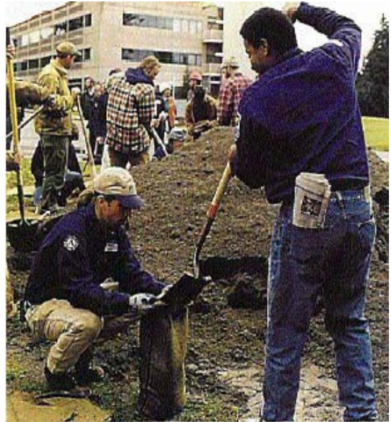
Figure 13.1 This two-person team is positioned properly for sandbag filling
