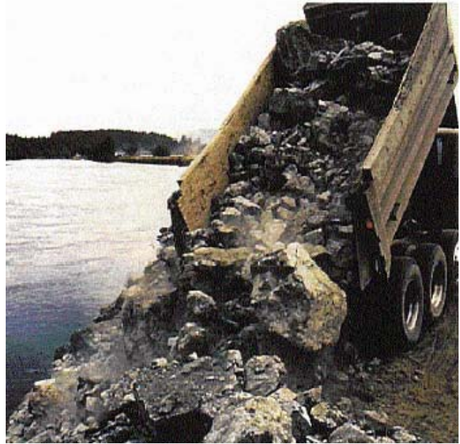
Figure 13.8 Placement of rock riprap. Careful use of an excavator may allow for more accurate placement than is shown above.
