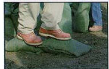
Place each succeeding bag tightly against and partially overlapping the previous one. Compact and shape each bag by walking on it.
