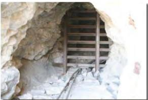
Above is the opening that had been sealed 3 times with 3 different methods. All of which were vandalized. This closure is a bat gate and was erected to allow bats to come and go from the mine shaft.
