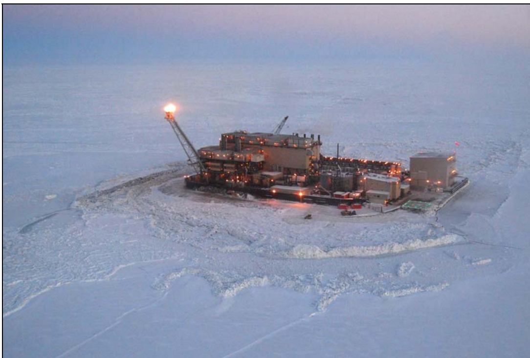
Plate 2. 8-m Ice Pile-Up on Northstar Production Island (November 27, 2012)
