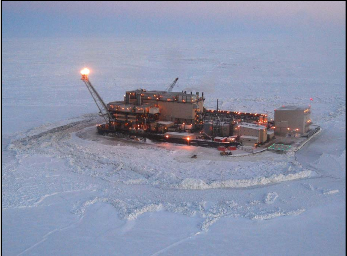
10-m Ice Pile-Up on Northstar Island (November 27, 2012)
