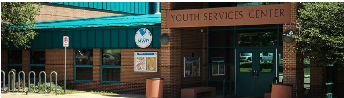
Youth Services Center, Category B MWR activity building at Fort Carson, Colorado.
