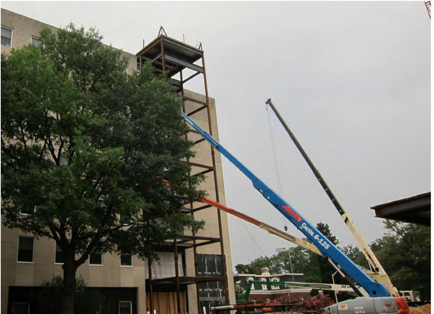
*New Sheridan elevator tower under construction*
