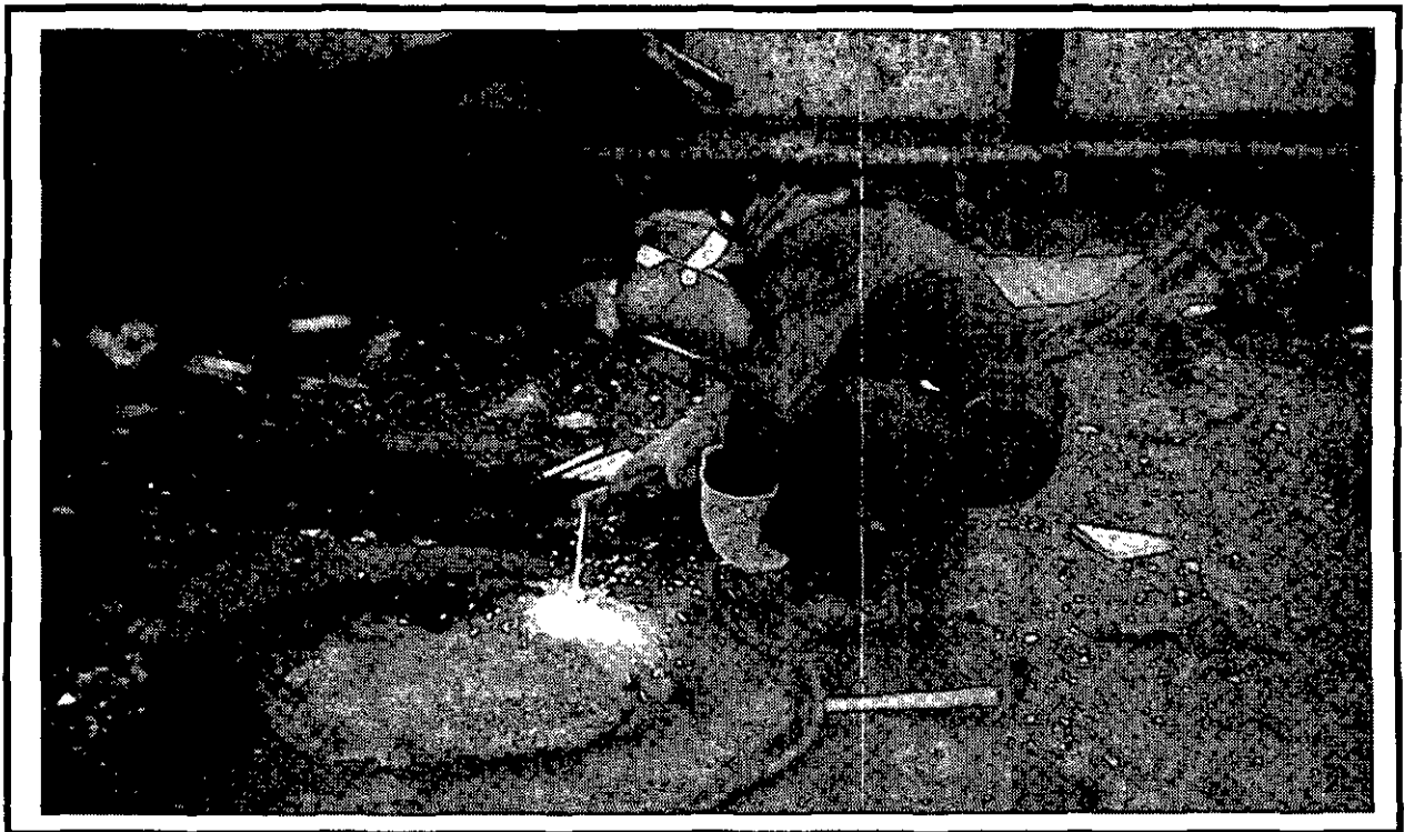
FIGURE 5-17. Welding Close Tank Tops.
