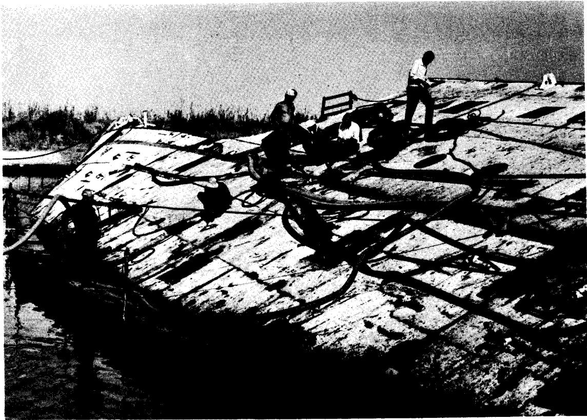
FIGURE V-15 Above-Water Cutting Operations on MECCA by SCA Burners
