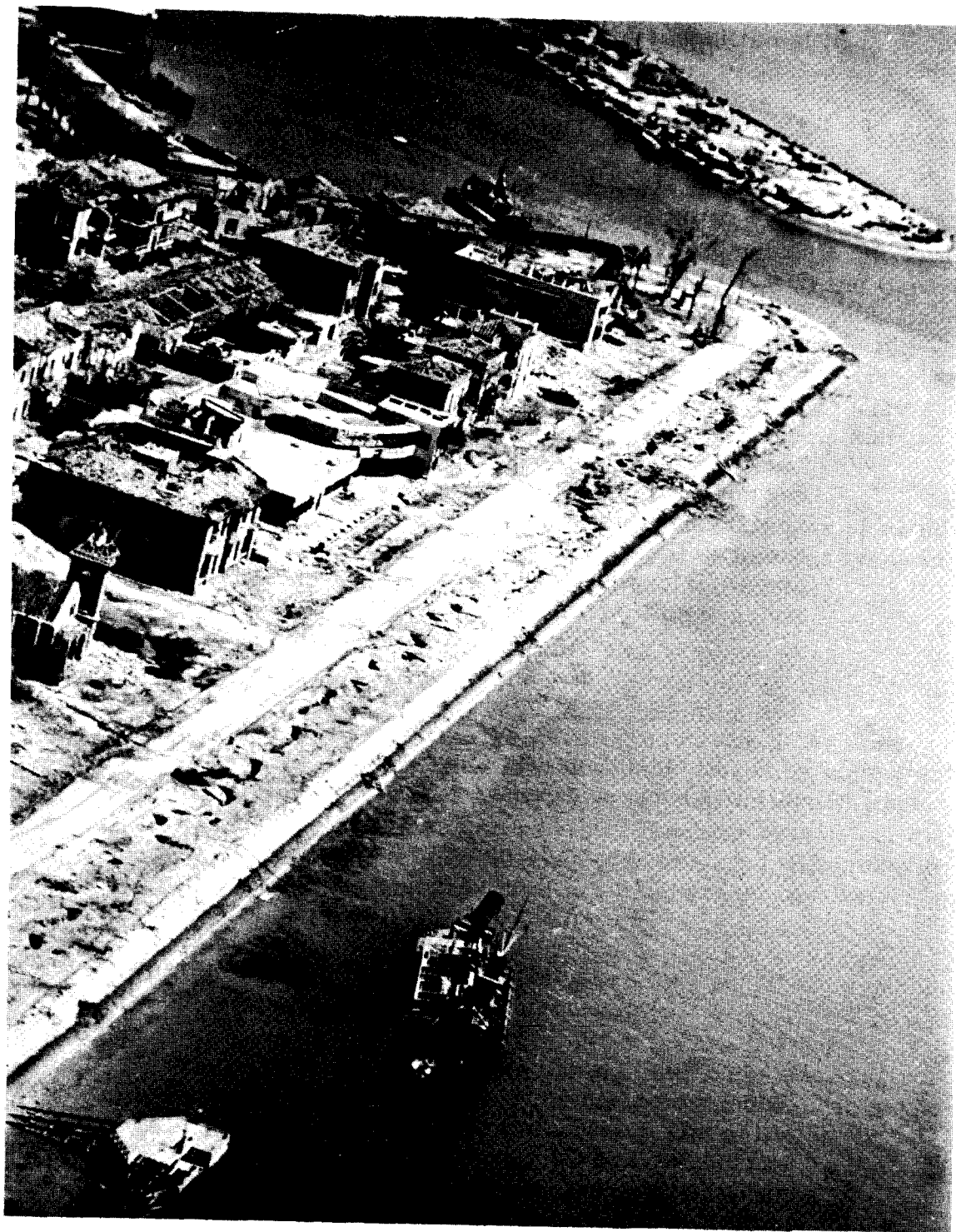
FIGURE III-4 Southern Entrance to Canal Showing Characteristic Port Taufiq Devastation
