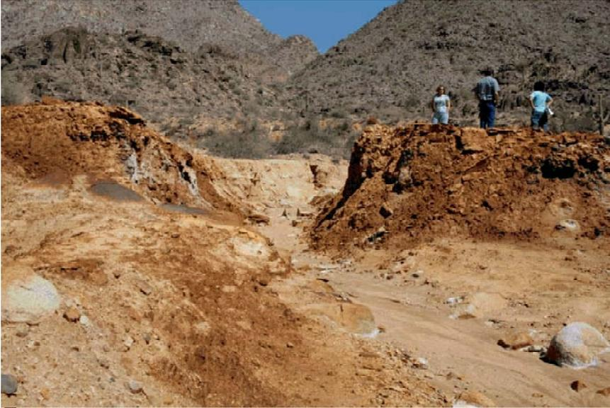
Massive tailings pile at the Antler Mines is being washed away.
