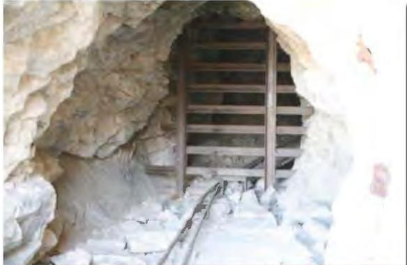
Above is the opening that had been sealed 3 times with 3 different methods. All of which were vandalized. This closure is a bat gate and was erected to allow bats to come and go from the mine shaft.
