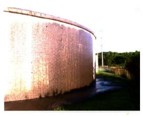
Dark staining on the walls and on the ground is raw sewage that has spilled over the sides of the tank. Bristol Plant employees then used a fire hose to wash this into a storm water grate that went directly into the Delaware River.
