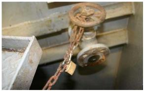
Locked overboard discharge valve
