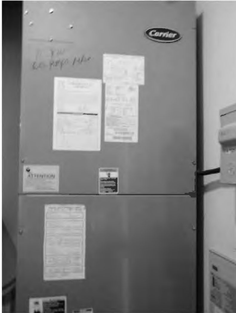
Photo 2—View of the three-ton air conditioning unit that is used for the upstairs of the house
