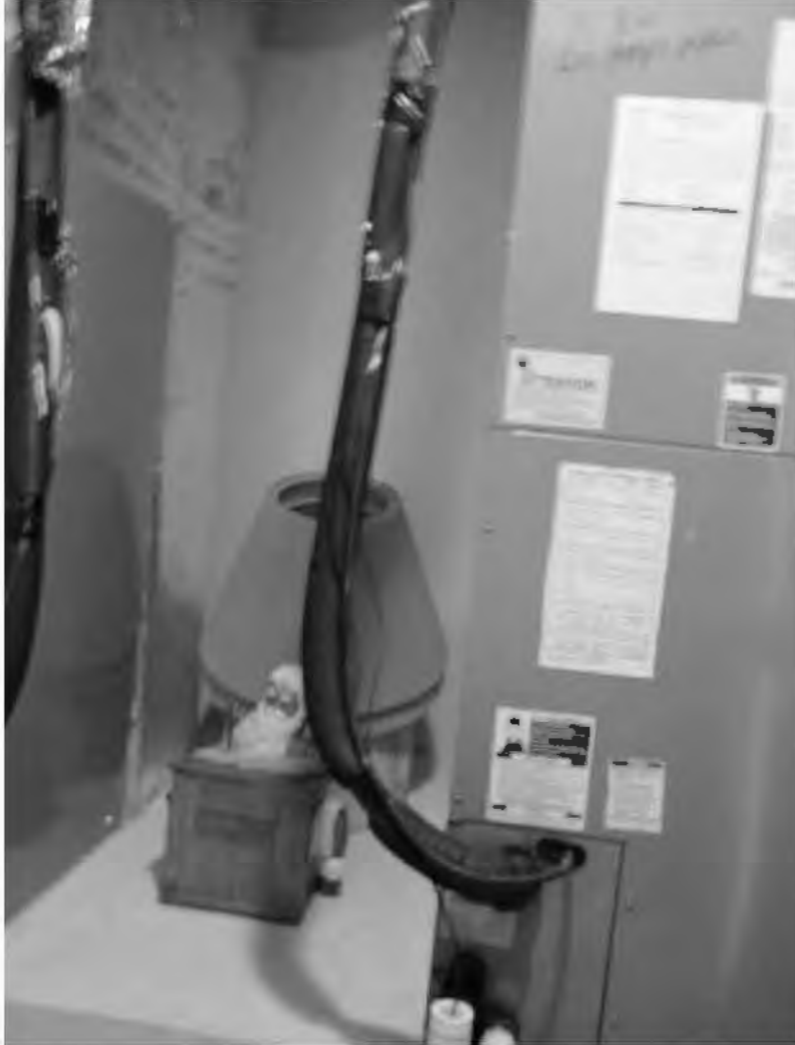
Photo 3—View of the copper wire that runs alongside the air conditioning unit that has turned black
