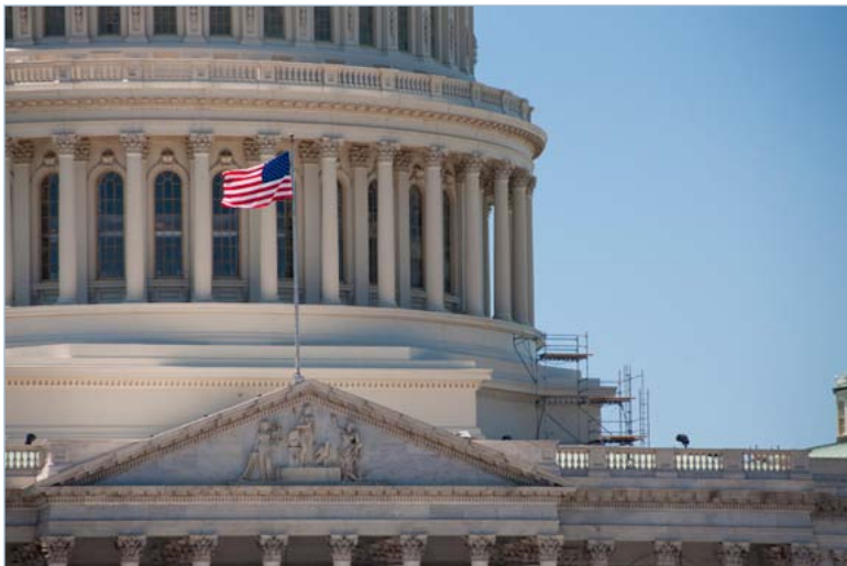
Scaffolding begins to rise on the northeast corner of the U.S. Capitol dome for a two-year restoration project. Learn more about the repairs at www.aoc.gov/dome/project-overview .
