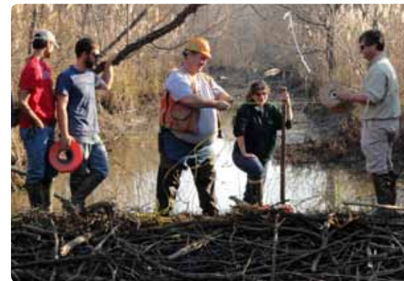
Standing atop a beaver dam, Wildlife Services’ (WS) Johnny Carter (center with hard hat) shows students how to string wire to detonate charges for dam removal. WS State Director Kris Godwin (right of Carter) watches the preparations.
