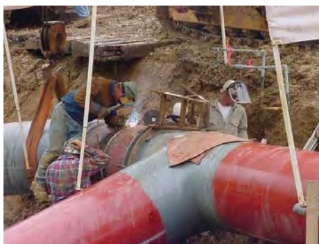
Williams-Transco engineers weld new 36" internal inspection device receiver to natural gas pipeline.
