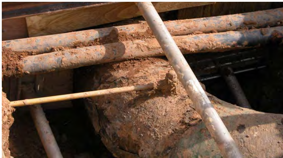
Damage to pipelines resulting from a crowded underground infrastructure is a major problem pipeline operators and regulators continue to face. The photo above shows an operator's discovery of newly installed fiber optic lines directly over natural gas pipeline.
