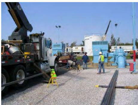
Emergency crews work to connect one of several mega-watt electrical generator trailers to meet the supplemental power requirements needed to restore operations at Colonial Pipeline and Plantation Pipeline pumping stations, storage tanks, and truck loading terminals in Collins, Miss.
