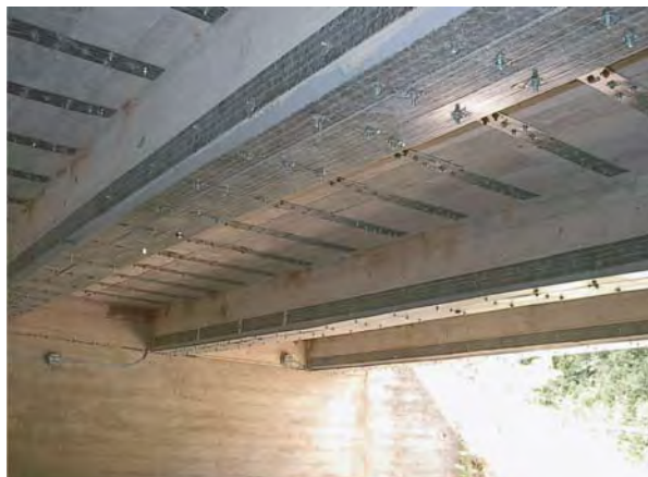
Deck and girders of a bridge strengthened with MF-FRP system.
