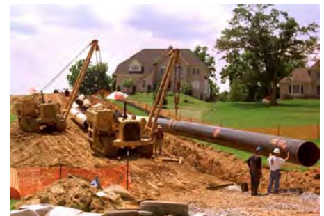
Contractors replace high-pressure pipeline in right-of-way recently encroached upon by new community.
