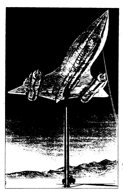
Radar testing of A-12 mockup
