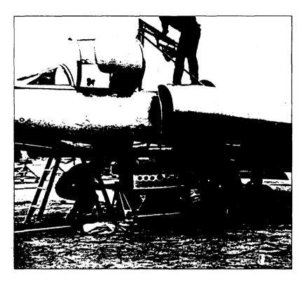
A-2 camera being installed in U-2
