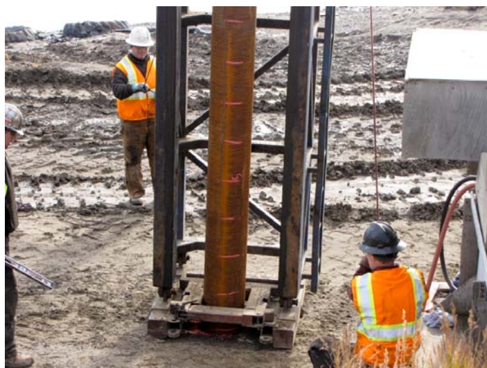
Driving piling into the ground. Piling provides anchorage for future mooring point.
