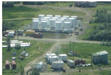
Newly Installed Bulk Fuel Tanks
