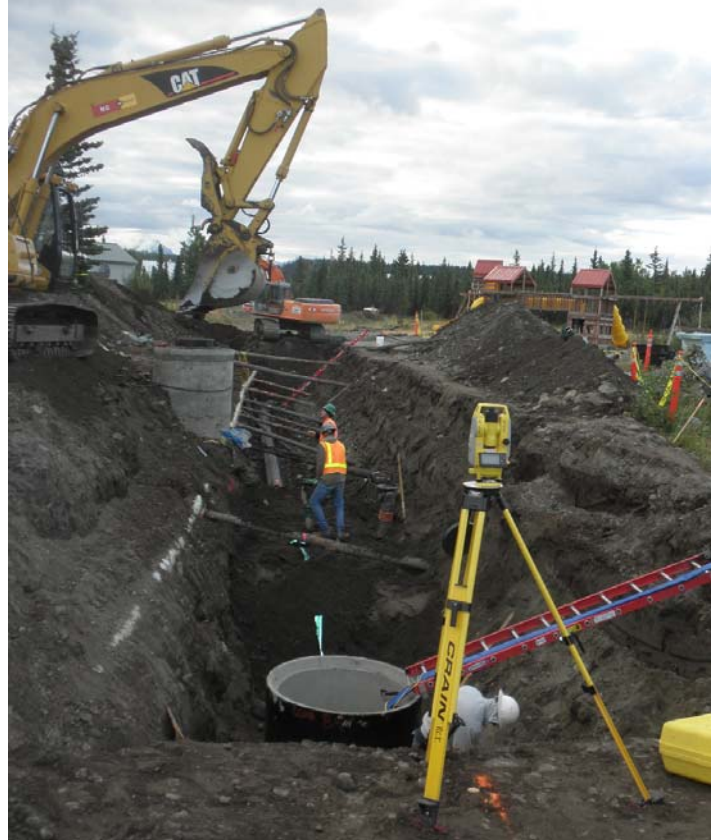
Digging ditch in Gulkana, preparing to lay water and sewer pipes. See additional project information in Section 3 of this report.
