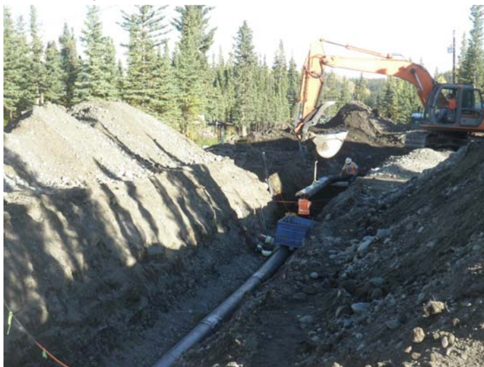
Backfilling ditch after water and sewer pipes have been laid.
