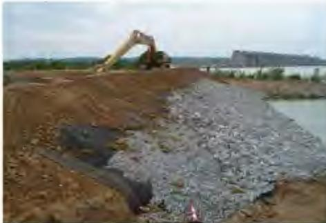
The "Long Stick" backhoe used to excavate first 80 feet of the soil-cement-bentonite slurry wall. The superstructure of the Smithland Dam is visible to the right.
