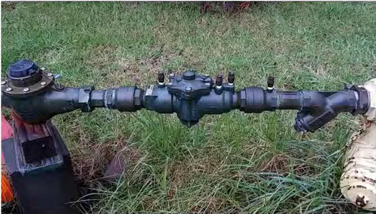
Figure 5. An example of the backflow preventers at HAVO. Source: OIG.
