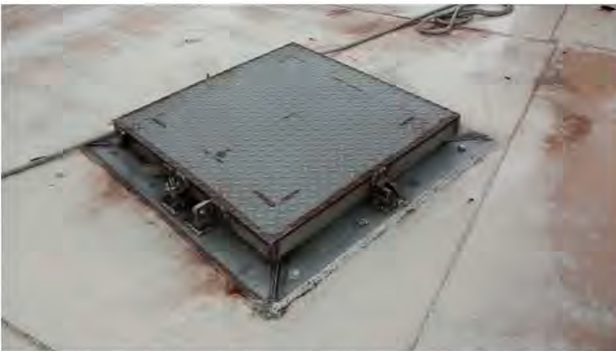
Figure 6. An access hatch sealed with silicone (visible on the lower right edge of the hatch's frame). Source: OIG.
