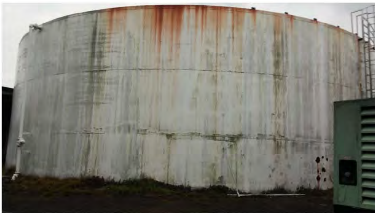
Figure 1. Corrosion on the exterior of a water storage tank. Source: Office of Inspector General (OIG).
