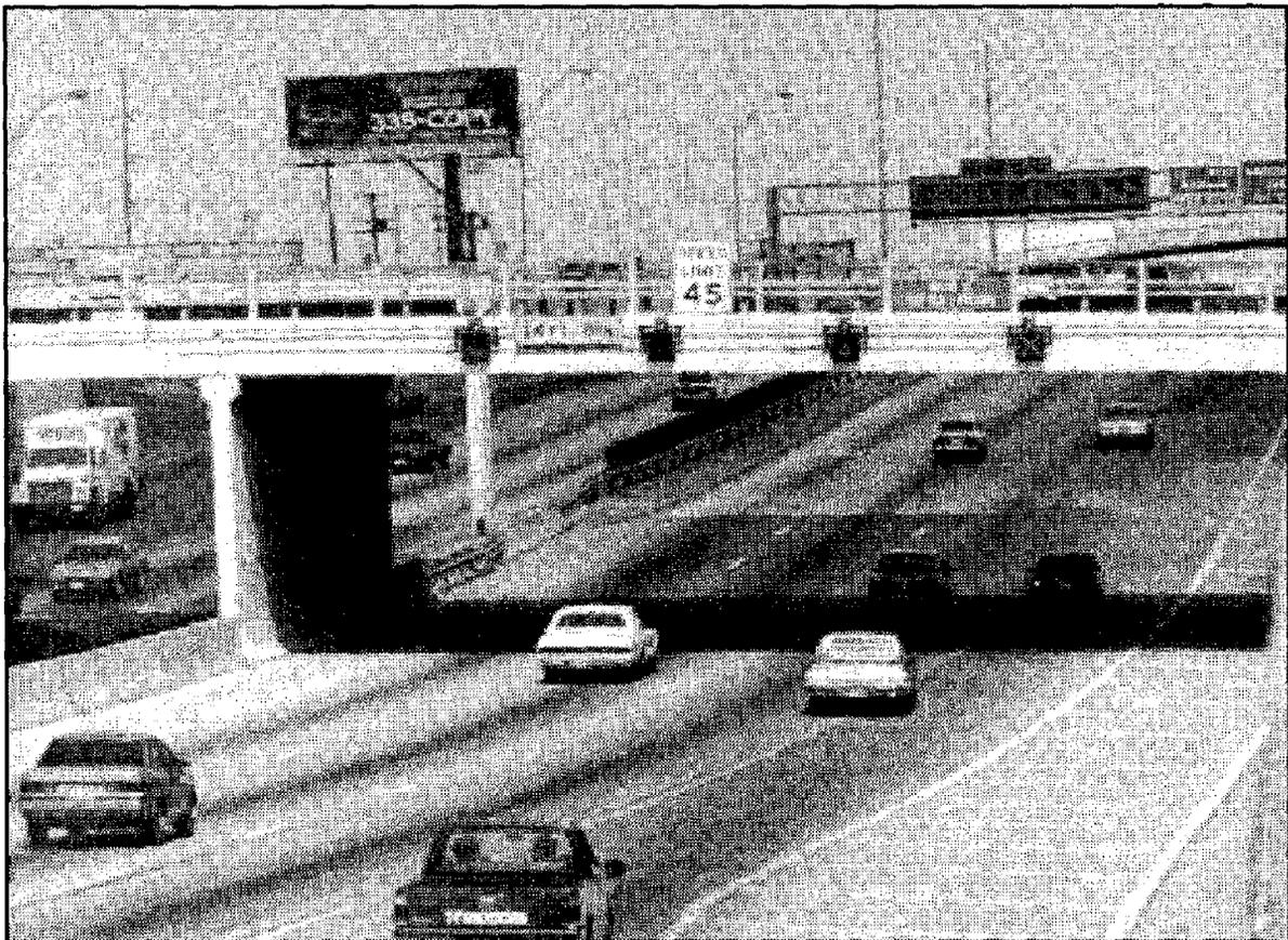
**Figure 4-3. Typical Freeway Lane Control Signal.**
