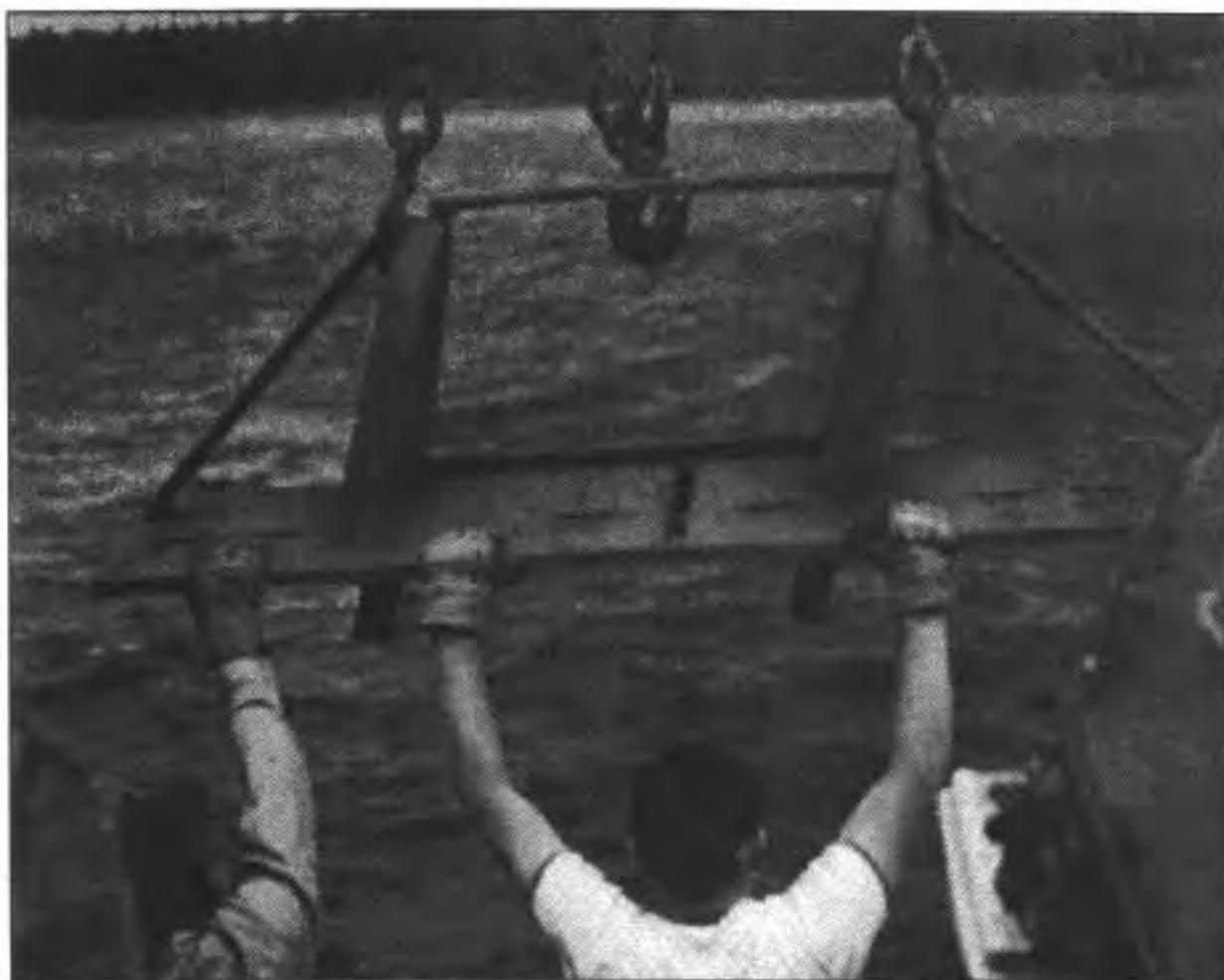
Figure 3-15A. Lift Pad Being Lowered into Place.
