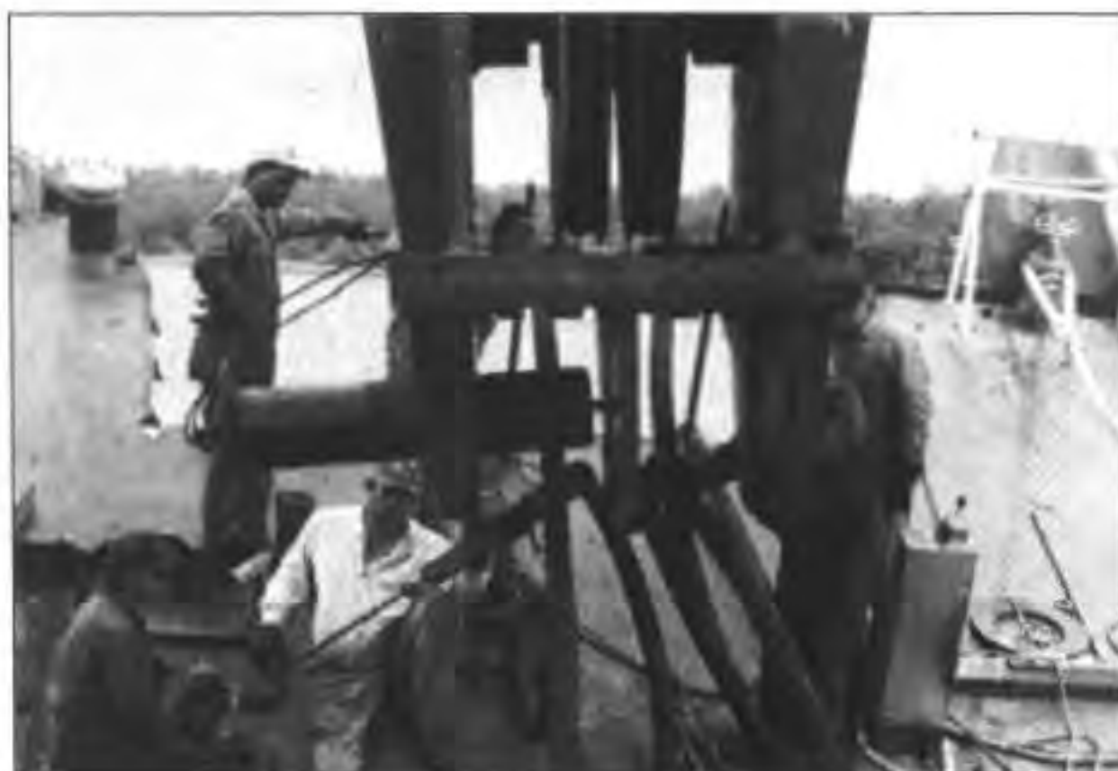
Figure 3-18. Lifting Pin Set to Capture Sling.
