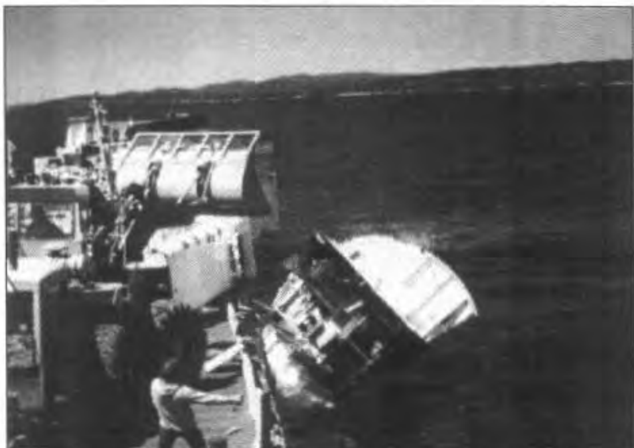
Figure 3-23. Superstructure Being Pushed Overboard at Disposal Site.
