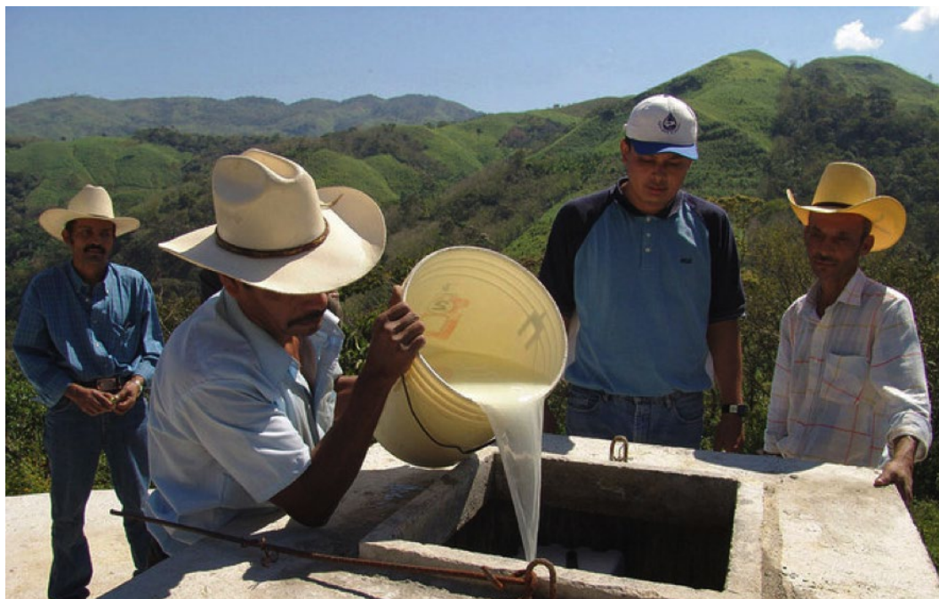
An engineer from Agua para el Pueblo, in Honduras, “teaches Agua Caliente’s water committee about maintenance, including the correct amount of chlorine to make the water safe and how to test the chlorine content weekly.”
