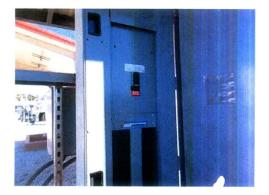
The existing main electrical switchgear will not require upgrading for the Phase 1 solar system. We recommend installing a reverse power relay(s) at the existing transformer. The inverter output over-current protection is via circuit breakers at the PV unit subsystem. These breakers will be lockable and serve as the owner's isolating disconnecting means. The utility isolating disconnect will be at the new PV unit subsystem and be separate and lockable.
