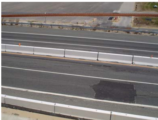
P6/7: North Roadway Approach Embankment – Surcharge placement has been completed. Surcharge elevation is at 51 ft. The embankment is currently being left to consolidate/settle. Once sufficient settlement has occurred, the additional surcharge will be removed, the drainage system will be installed, and the concrete facing on the MSE walls will be installed. There has been 4 months of surcharge completed, with 4 months more anticipated.
