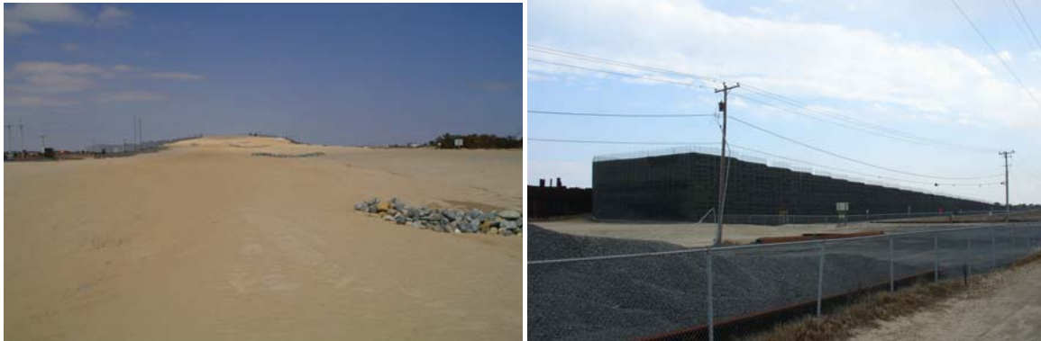
P4/5: South Roadway Approach Embankment – Surcharge placement was completed on February 20, 2007. Surcharge elevation is at 51 ft. The embankment is currently being left to consolidate/settle. Once sufficient settlement has occurred, the additional surcharge will be removed, the drainage system will be installed, and the concrete facing on the MSE walls will be installed. There has been 2 months of surcharge completed, with 6 months more anticipated.
