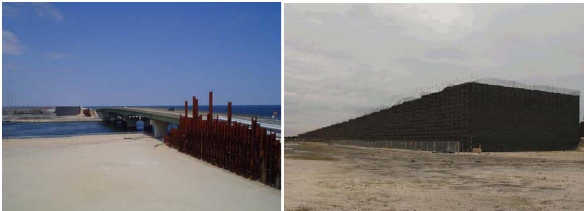
P6/7: North Roadway Approach Embankment – Surcharge placement has been completed. Surcharge elevation is at 51 ft. The embankment is currently being left to consolidate/settle. Once sufficient settlement has occurred, the additional surcharge will be removed, the drainage system will be installed, and the concrete facing on the MSE walls will be installed. There has been 4 months of surcharge completed, with 4 months more anticipated.
