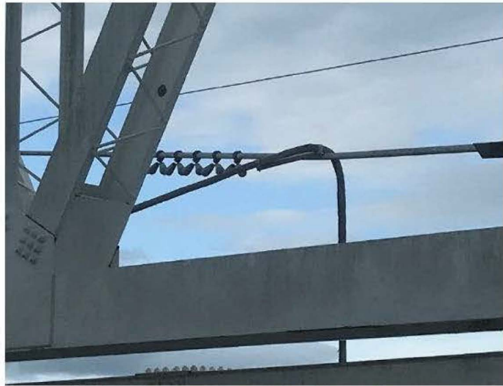
Figure 7. Failed cable draped over T12 auxiliary cable. Photo from AO.
