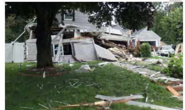
Figure 48. Only remnants of this house remained after the explosion and fire in Merrimack Valley, Massachusetts, in which 1 person was killed and 22 people were severely injured.
