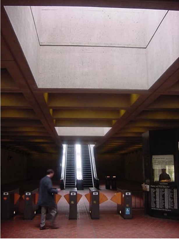
Figure 22: Skylight wells
