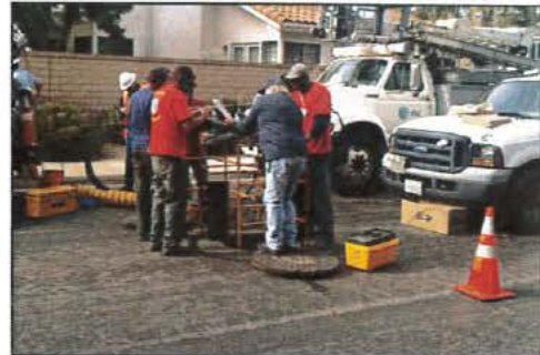
Figure 4 – (U) Repair of severed fiber optic lines in Del Mar, CA (SOURCE: NBC News)
