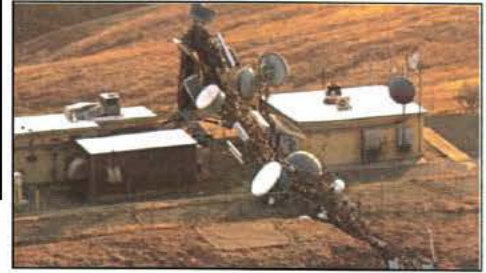
Figure 4 – (U) Collapsed public safety communications tower near San Ramon, CA (SOURCE: KTVU USPER )
