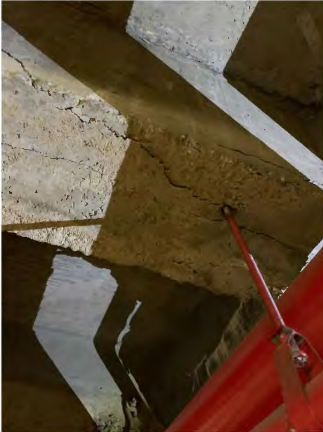
Picture 16: Deteriorated Concrete Waffle Slab (Cracks & Delamination)
