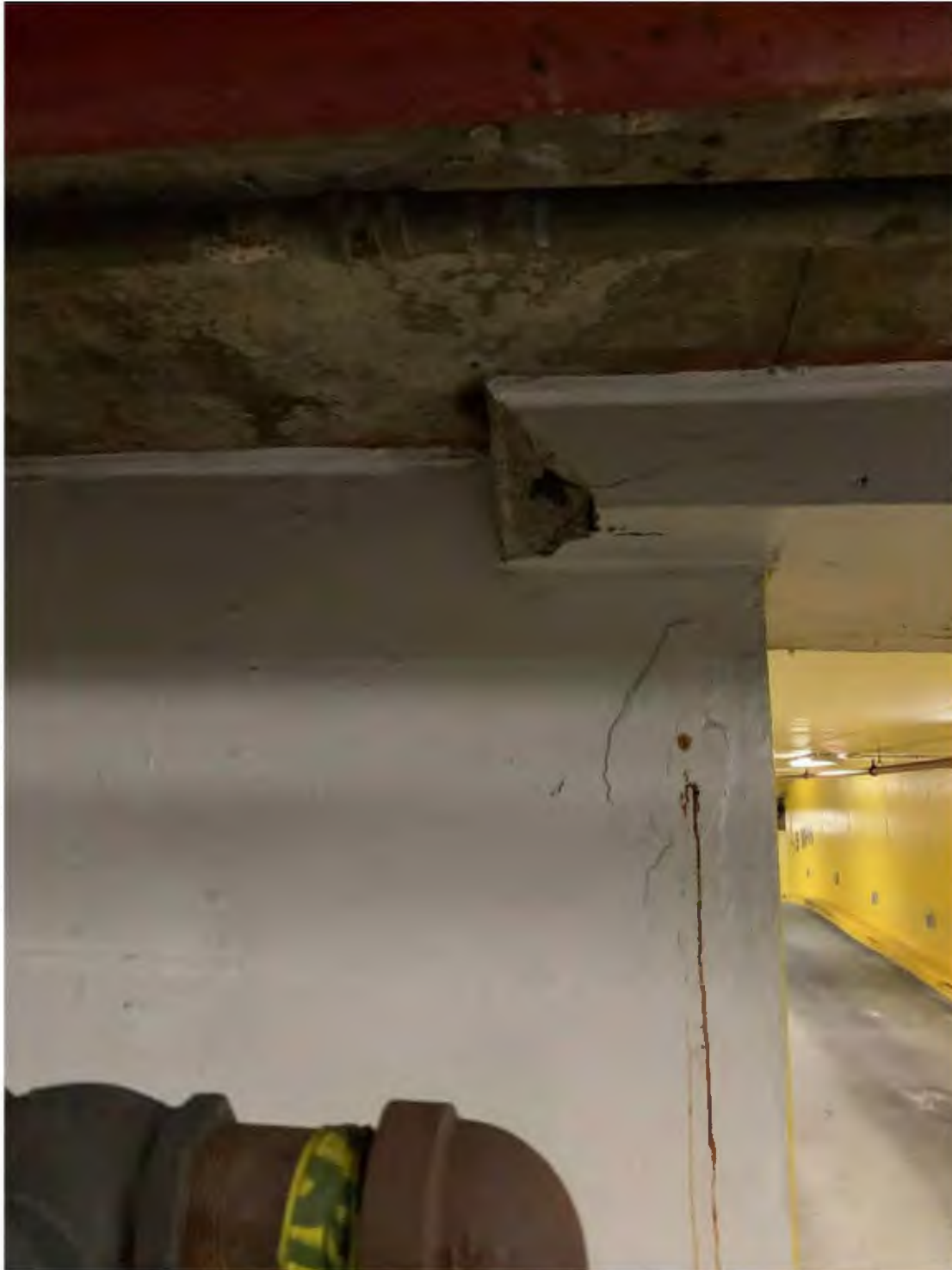
Picture 1: Cracks in Concrete Wall
