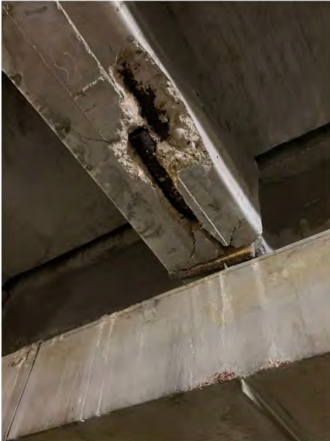
Picture 17: Deteriorated Concrete Waffle Slab (Cracks & Delamination)
