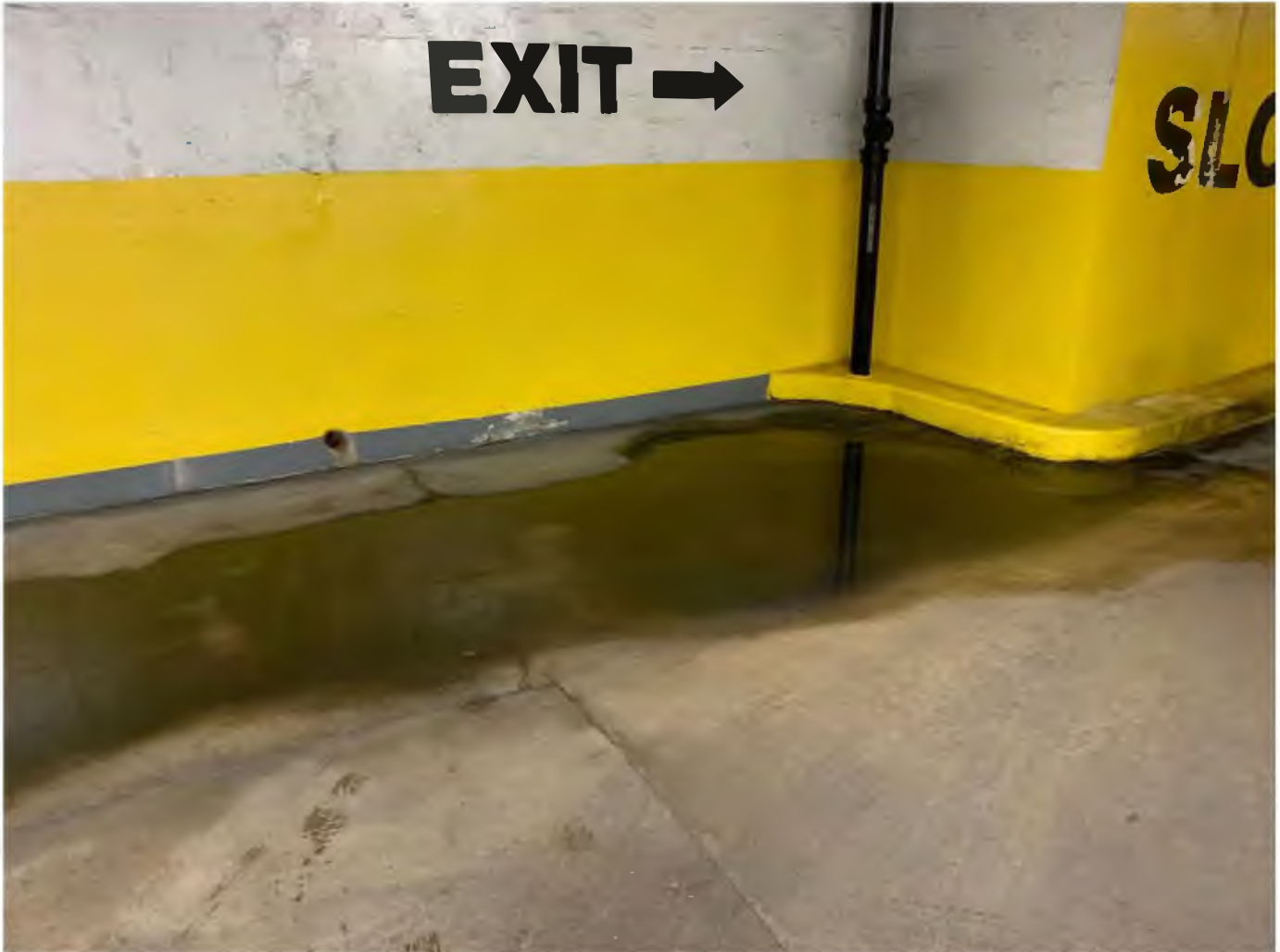
Picture 19: Large water ponding at Level-C, bottom ramp, that is not properly draining due to no slope in the slab.
