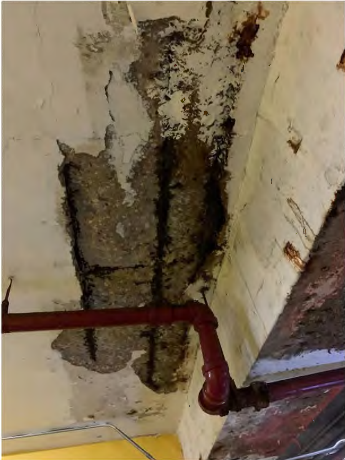
Picture 11: Deteriorated Concrete Beam
