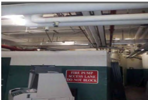
C1011 - Fire Pump Room - Add Rated Separation 1
