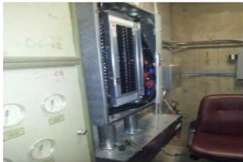
D5012 - Electrical Equipment Covers Missing - Replace
