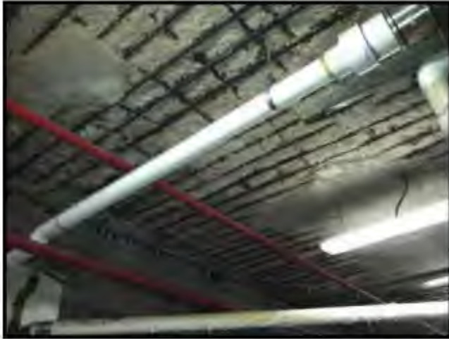
A2020 - Structural Slab Spalling - Repair
