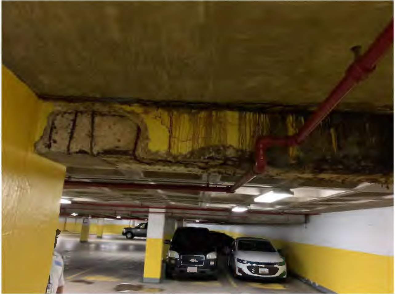
Picture 9: Deteriorated Concrete Beam
