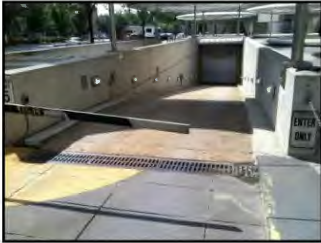
B1015 - Garage Ramp Falloff Protection - Add
