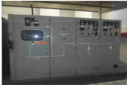
D5011 - Medium Voltage Primary Service Switchgear - Replace
