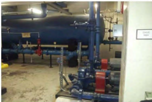
D2020 - Restroom Water Pressurization System - Replace 2
