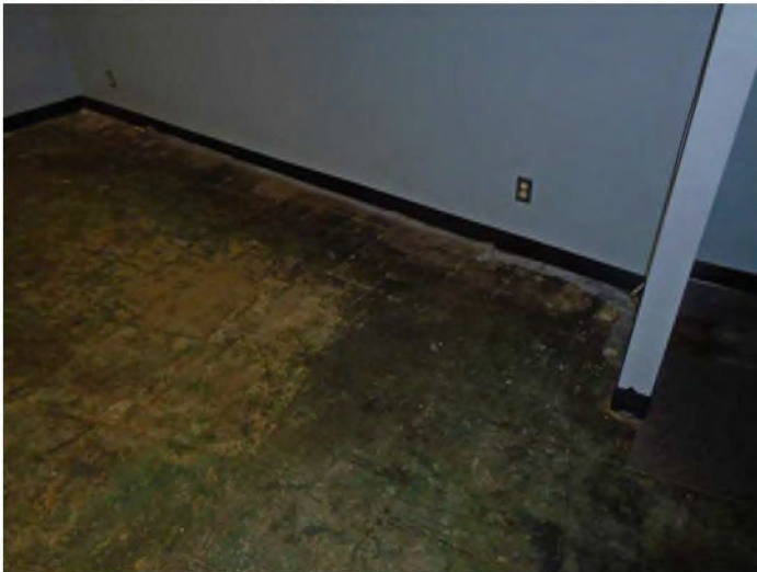
Photo Seal-5: Water damage in Room B182
