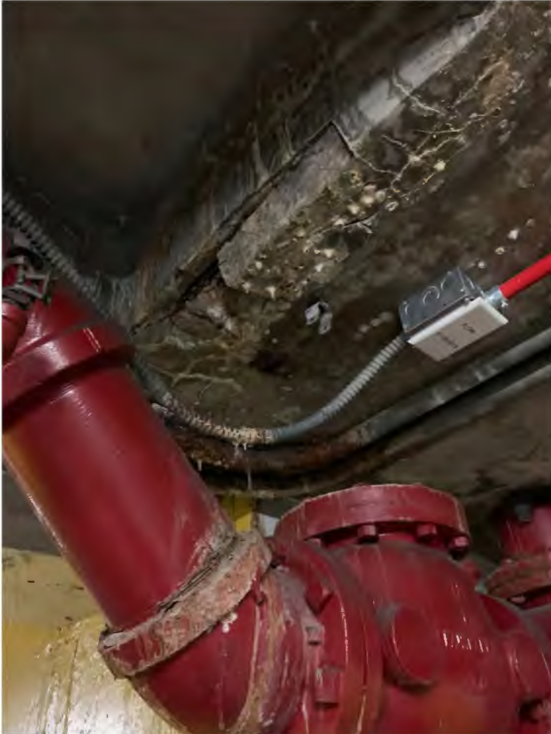
Picture 7: Deteriorated Concrete Beam
