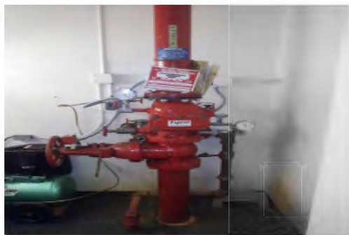
C1011 - Standpipes Not Enclosed - Add Rated Separation
