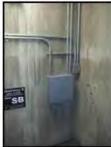
C1011 - Panels and Conduits Exposed in Stairs - Add Rated Separation
