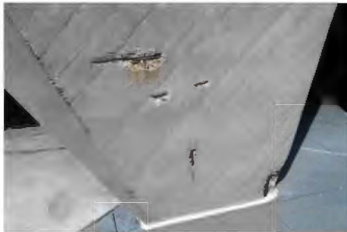
B2011 - Exterior Tree Columns Spalling - Repair
