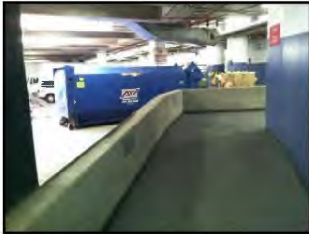
C2010 - Loading Dock Handrails - Provide Guards
