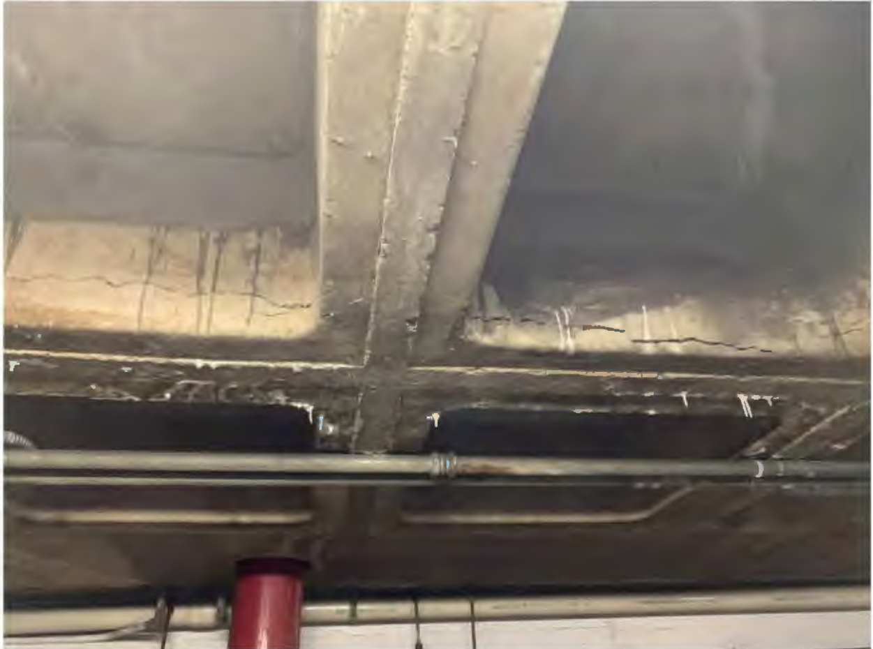
Picture 14: Deteriorated Concrete Waffle Slab (Cracks & Delamination)
