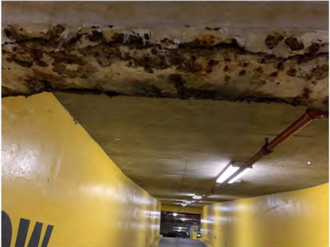
Picture 10: Deteriorated Concrete Beam
