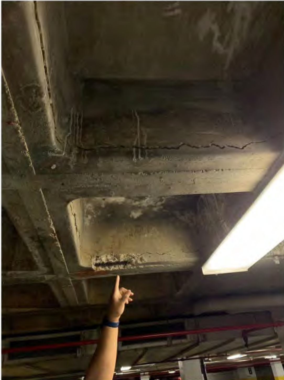
Picture 15: Deteriorated Concrete Waffle Slab (Cracks & Delamination)
