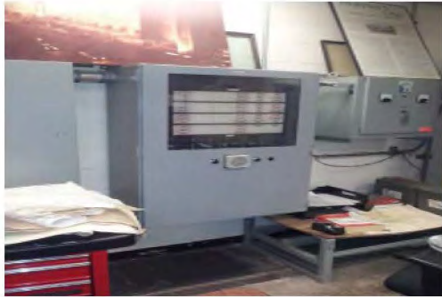
D5037 - Fire Alarm System - Replace 2
