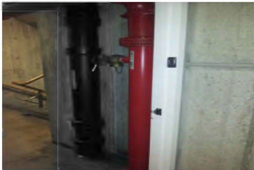
C1011 - Exposed 8 StormSewer Lines in Stairs - Add Rated Separation
