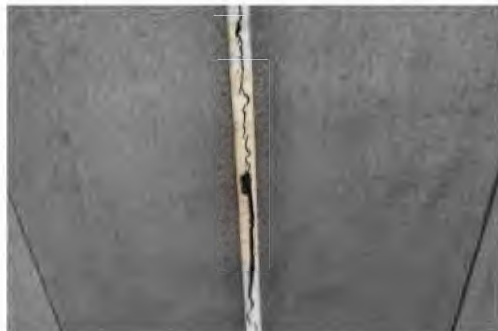
B2011 - Exterior Wall Expansion Joint - Replace
