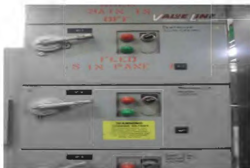
D5012 - Misc Electrical Equipment Motor Control Centers - Replace 2
