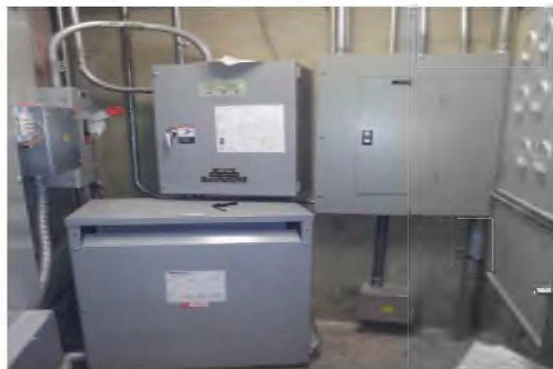
D5012 - Electrical Panels Clearance- Modify
