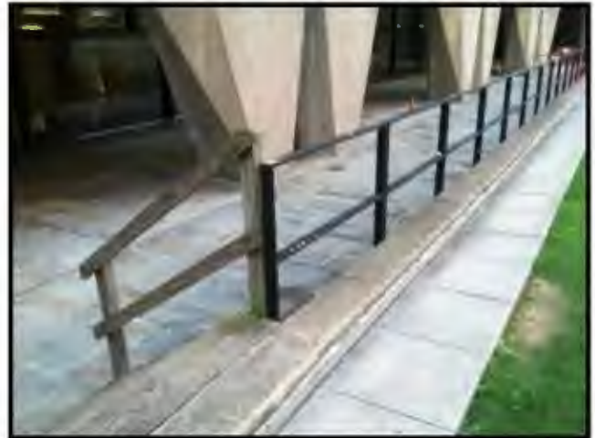
B1015 - Exterior Plaza Handrail Falloff Protection - Add
