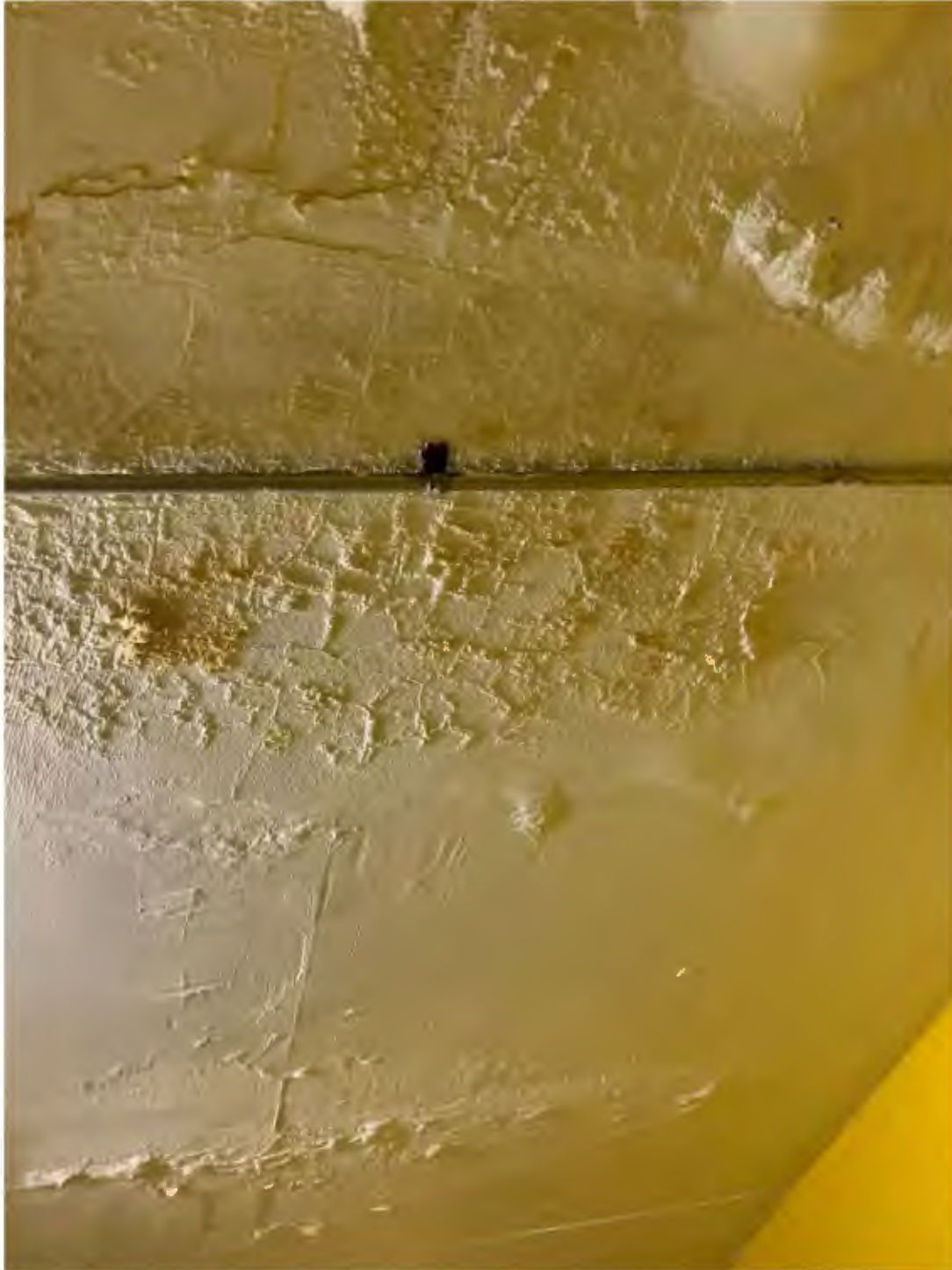
Picture 13: Deteriorated Concrete Slab at Ramp (Efflorescence & Delamination)
