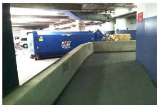
C2010 - Loading Dock Handrails - Provide Guards
