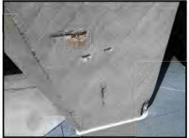
B2011 - Exterior Tree Columns Spalling - Repair
