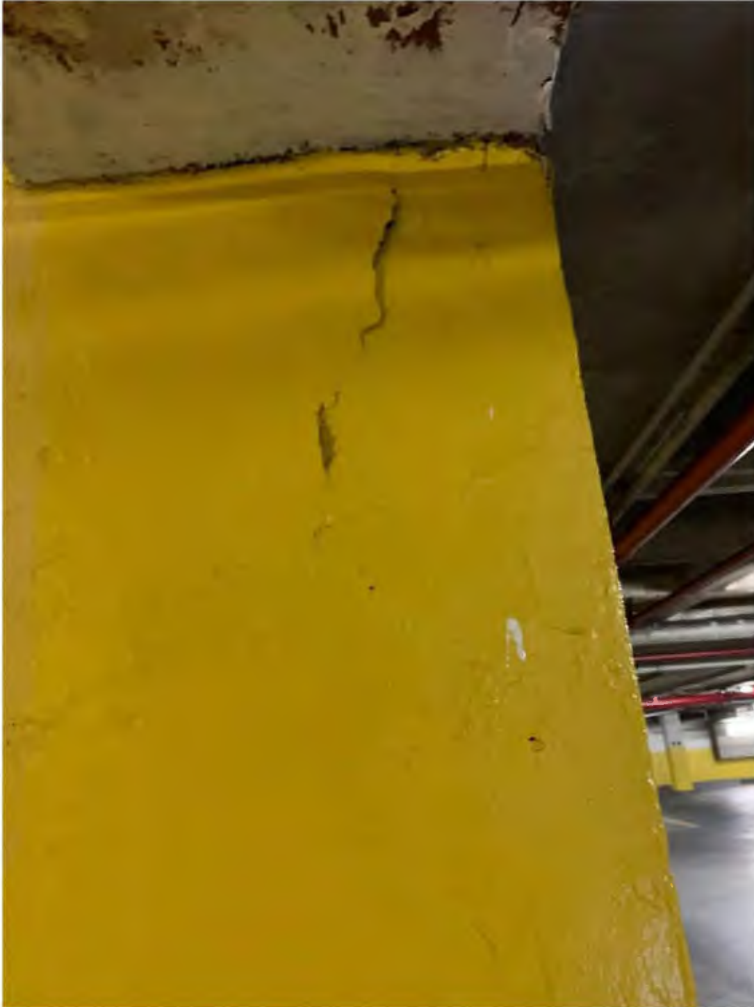
Picture 3: Cracks in Concrete Wall
