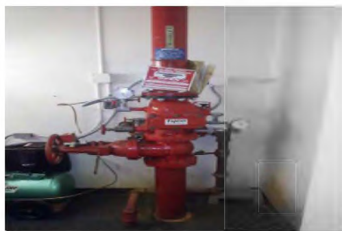
C1011 - Standpipes Not Enclosed - Add Rated Separation
