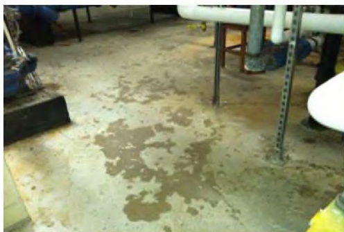
C3020 - Concrete Floor - Reseal
