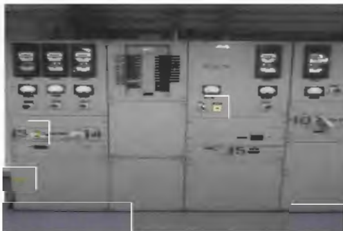
D5012 - Elevator Electrical Switchboard - Replace
