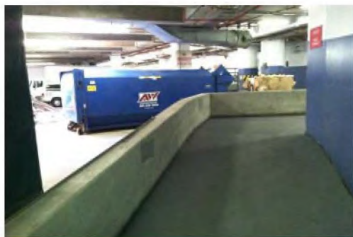
C2010 - Loading Dock Handrails - Provide Guards
