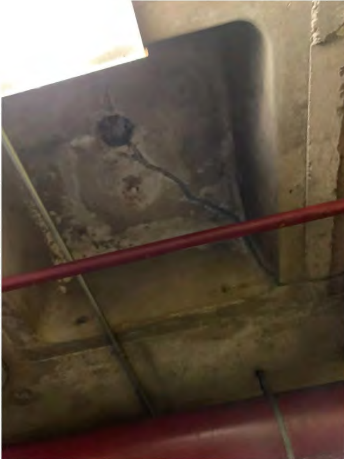
Picture 18: Deteriorated Concrete Waffle Slab (Cracks & Delamination)
