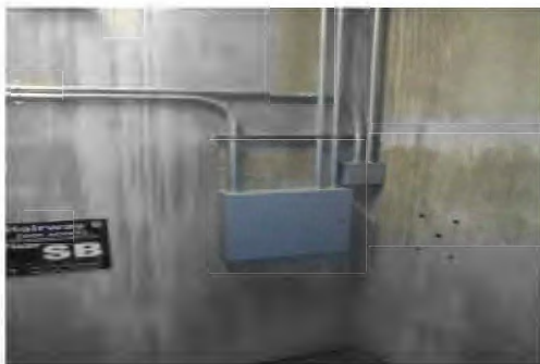
C1011 - Panels and Conduits Exposed in Stairs - Add Rated Separation
