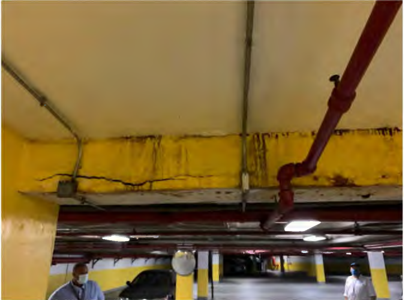
Picture 6: Deteriorated Concrete Beam
