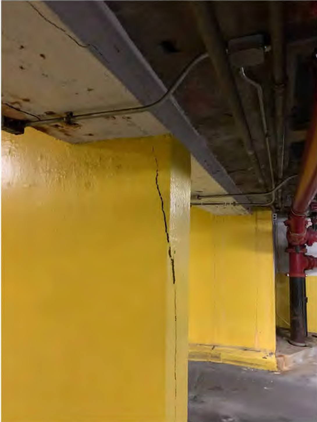
Picture 2: Cracks in Concrete Wall
