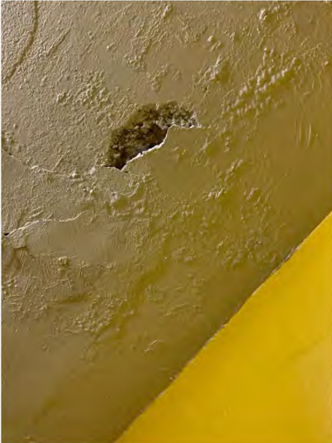
Picture 12: Deteriorated Concrete Slab at Ramp (Efflorescence & Delamination)
