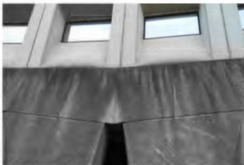
B2011 – Exterior Precast Sealant - Replace
