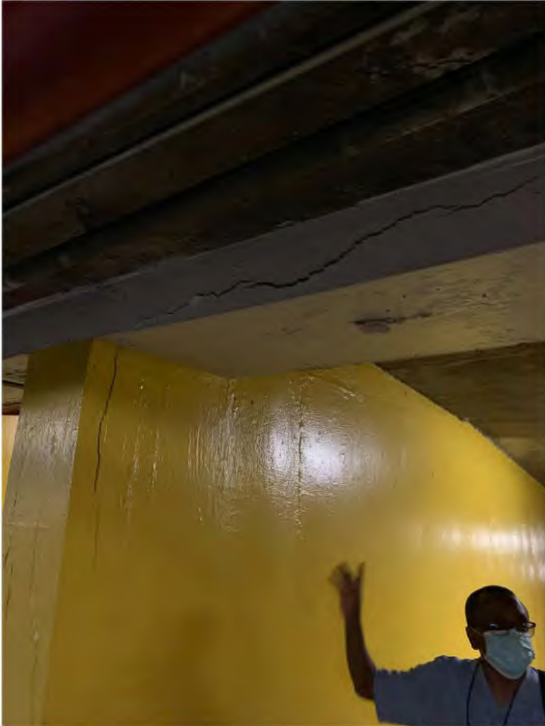
Picture 5: Cracks in Concrete Wall Beam Intersection
