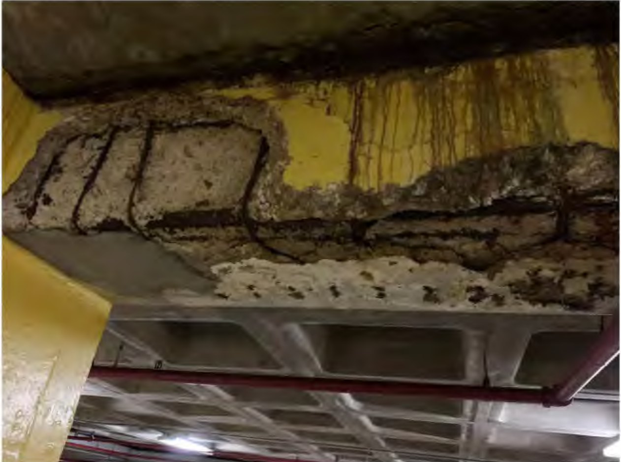
Picture 8: Deteriorated Concrete Beam
