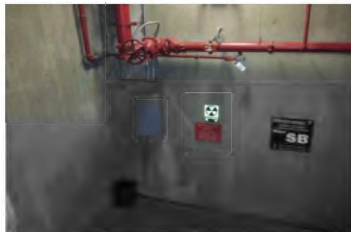
D4024 - Fire Hose Valve - Install
