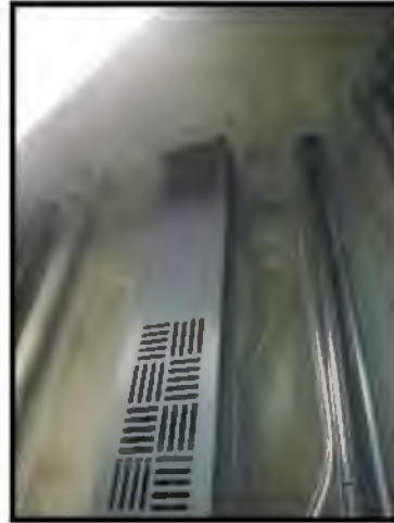
C1011 - Electrical Closet Shaft Opening - Add Rated Separation
