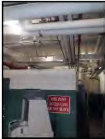
C1011 - Fire Pump Room - Add Rated Separation 1
