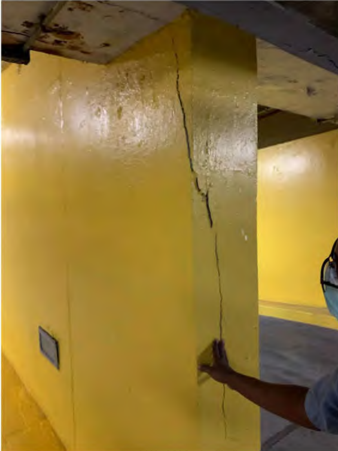
Picture 4: Cracks in Concrete Wall
