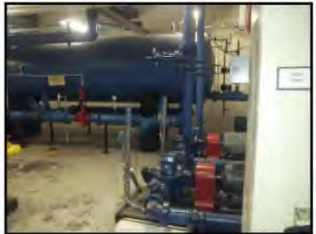
D2020 - Restroom Water Pressurization System - Replace 2
