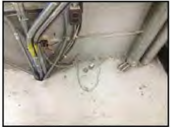
C1011 - Firestopping @ Floor Penetrations - Repair
