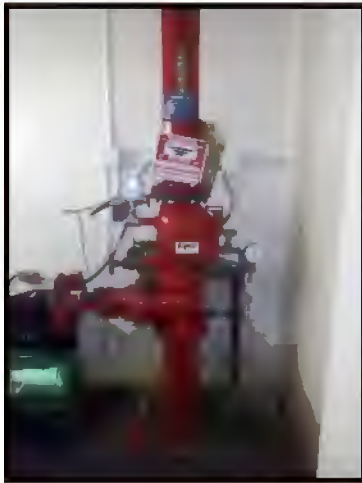
C1011 - Standpipes Not Enclosed - Add Rated Separation
