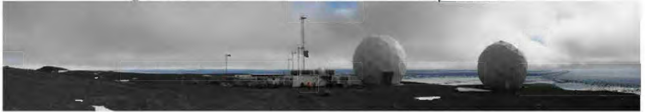
Figure 9: Black Island Communication Facility
