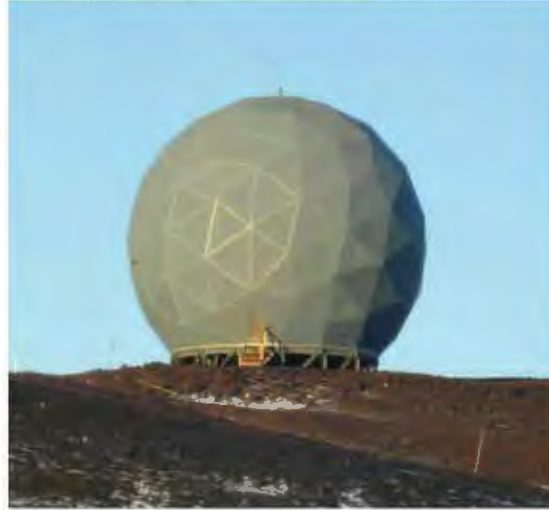
Figure 10: Telecom NZ 9m antenna at Arrival Heights
