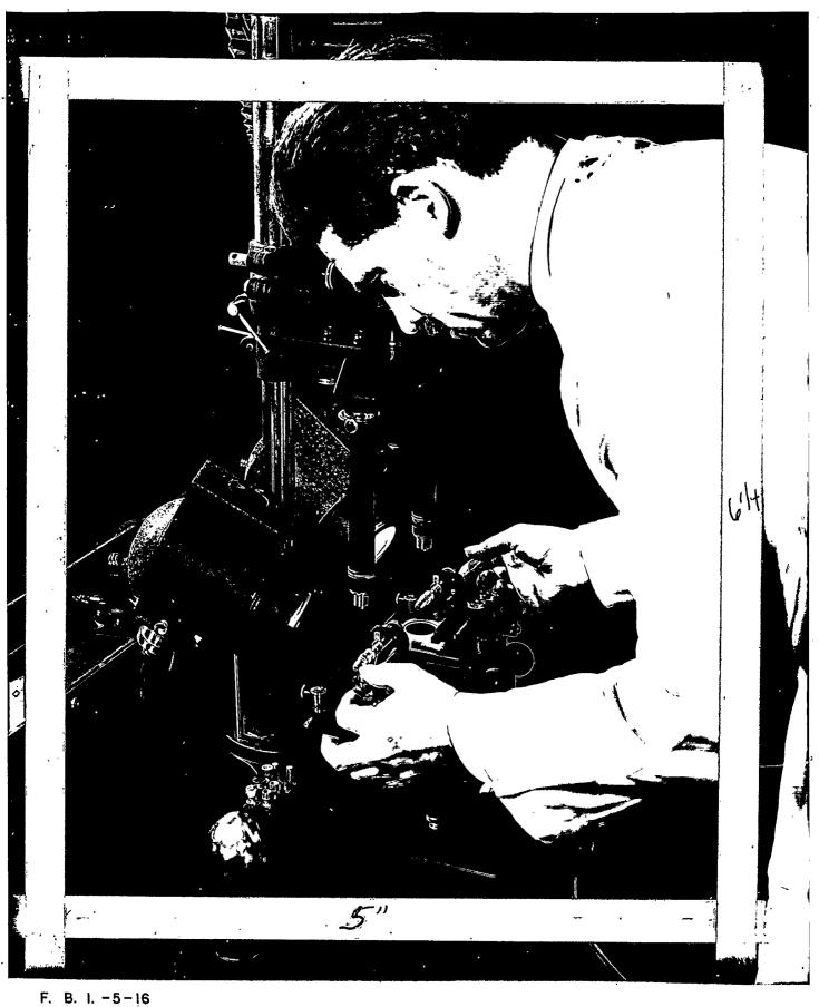
VIEWING A SUSPECT BULLET WITH A TEST BULLET THROUGH THE COMPARISON MICRO-SCOPE AT THE TECHNICAL LABORATORY OF THE FEDERAL BUREAU OF INVESTIGATION, UNITED STATES DEPARTMENT OF JUSTICE.
