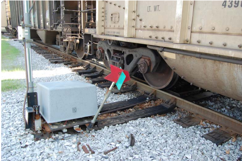
Switch box where the derailment occurred
