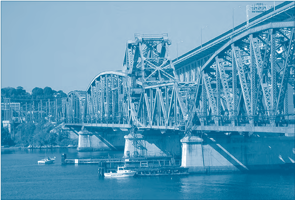
Slated to be rebuilt by 2008, the Thames River Bridge is a key transportation link on the route between New York and Boston. The bridge's bascule lift will be replaced with a vertical lift structure.
