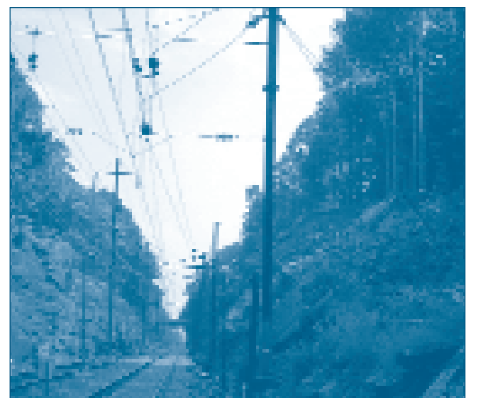
The clearing of the brush in Conewago, PA, is one segment of the 45 track miles on the Harrisburg Line that have been cleared at the direction of the Engineering department. This program has reduced the number of power outages and service failures by 20 percent since the spring.
