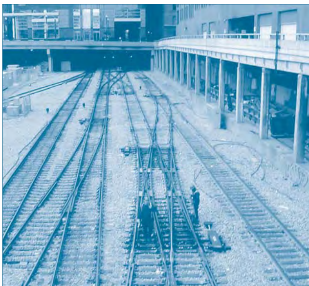
Signal Maintainers Victor Reap and John Vaughn inspect the newly installed N453A slip switch at the Lake Street Interlocking.
