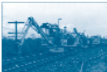
A tie gang, led by two tie cranes, works along a BNSF Oregon route.
