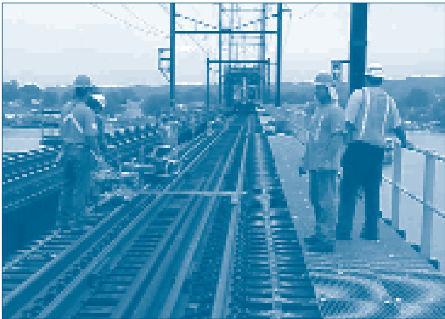
Track and structures production employees drill and install bridge tie spacing bars on the Susquehanna River Bridge, while the crane distributes materials to the site.
