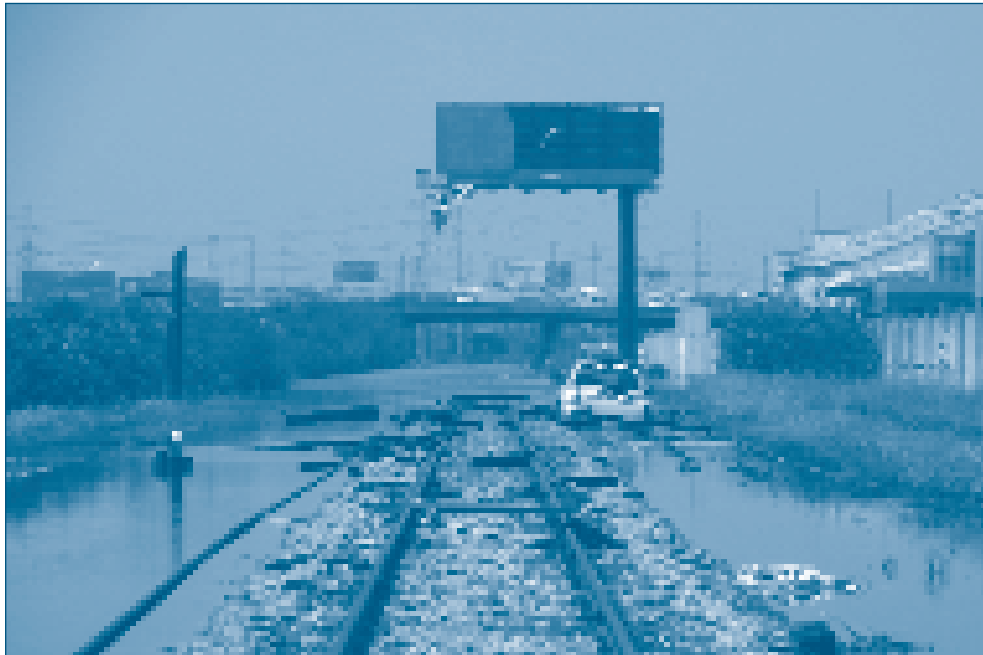
Heading north to Carrollton Junction, the tracks in the New Orleans Yard are washed out. Many of the signal components and switches were flooded as a result of Hurricane Katrina.
