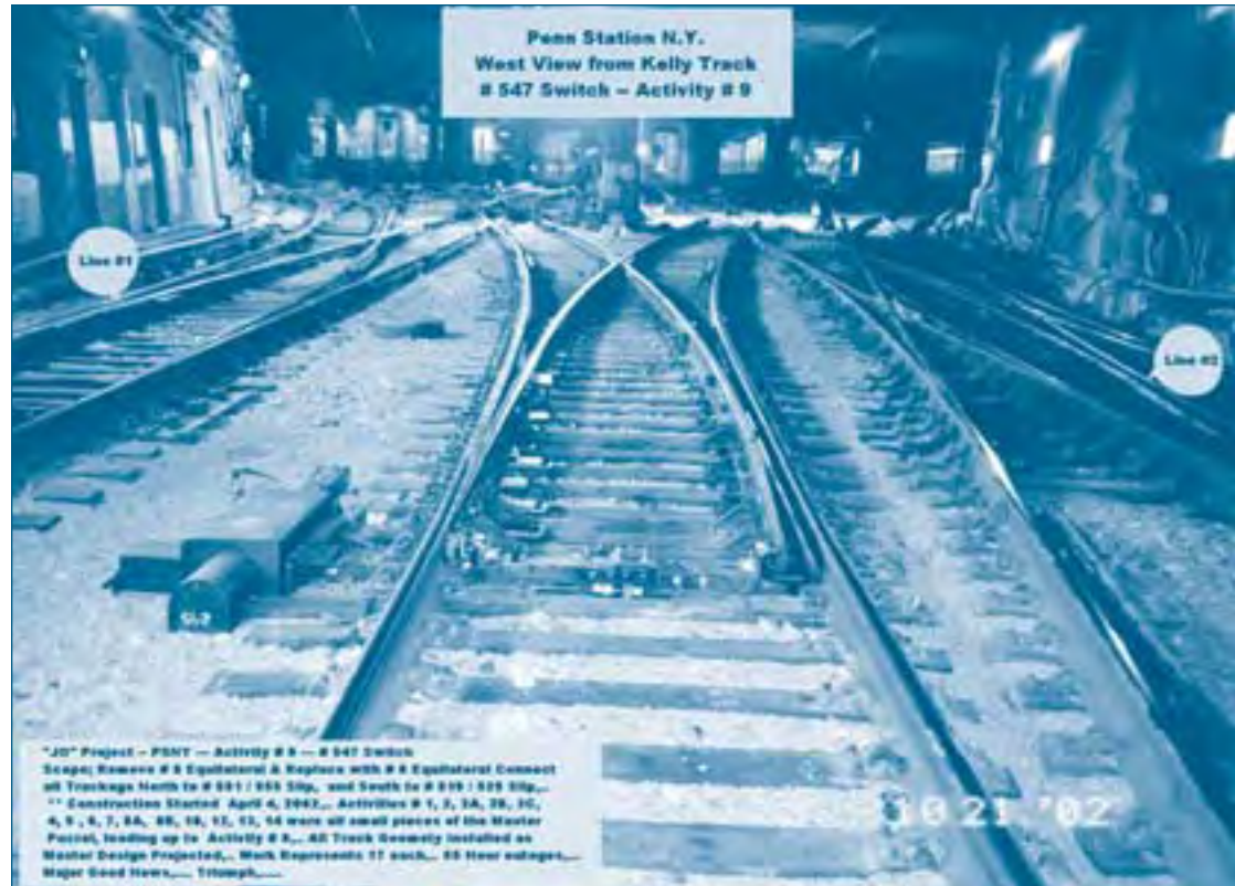
(Facing west into the station) The center switch could not be occupied at the same time as the switches on either side. To increase track usage in these locations, Amtrak started with track and switch changes extending to points fanning out near the train (whose rear car is visible).
