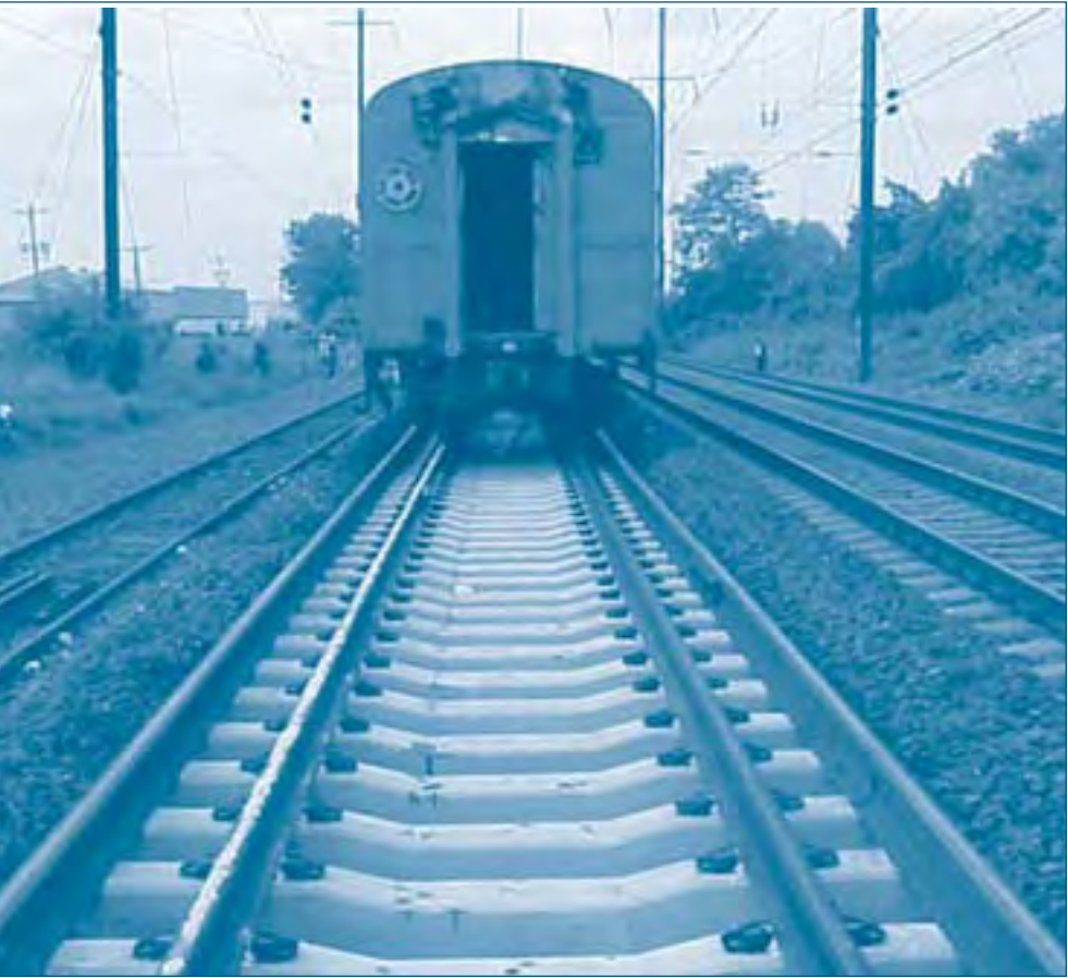
Clockwise from above: 1. The Ballast Cribber plows off ballast shoulder in preparation for TLM operation. 2. The TLM rail lining station, looking ahead at the complete material exchange. 3. The Pettibone swing and cart are used to cut out or add rail for proper thermal adjustment after the TLM has installed new ties. 4. Material exchange is complete, as the box car trails the end of the TLM. 5. New concrete ties and clips are seen in the foreground, while old wood ties are seen in the background.
