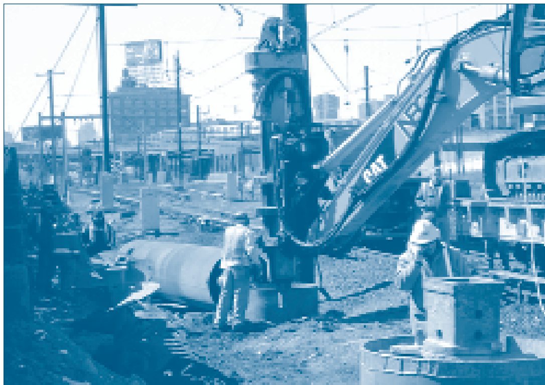
At New York's Sunnyside Yard, new catenary pole foundations are being drilled as work begins to accommodate additional tracks for the East Side Access project. The long-term project between Amtrak, the MTA, Long Island Rail Road and Metro-North will benefit commuter agencies and Amtrak by providing direct access to Grand Central Terminal for LIRR commuters and reduce congestion in the busiest railroad interchange in the country.
