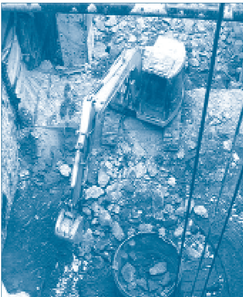
Demolition of the shafts of the Long Island City ventilation system reaches 40 feet below the ground.
