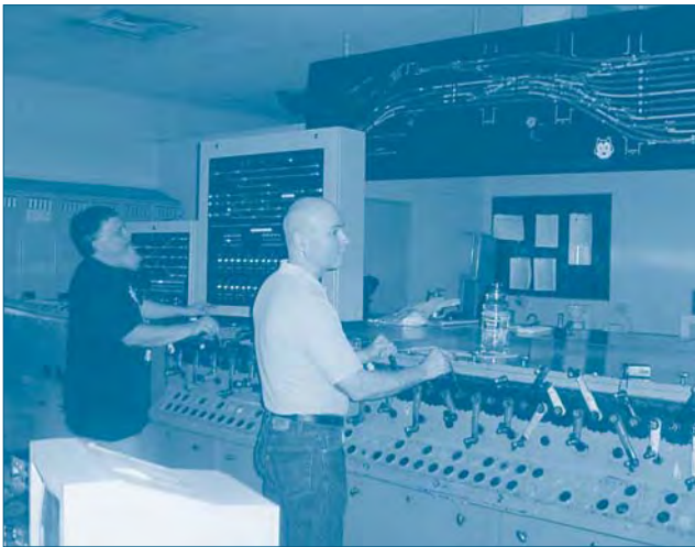
Inside the Lake Street Tower, Train Director Doug Mathew (right) guides a train by operating the old interlocking machine, while Steve Pivoney (left) lines up a train with the new signal panel, which is being used temporarily until the old interlocking machine is discontinued. Once the upgrade project is complete, both the old and new interlocking systems will be discontinued and train movement will be directed by a new computer-based microprocessor.
