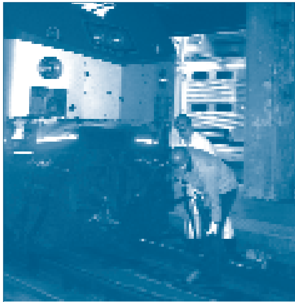
To conserve fuel and reduce emissions at Chicago Union Station, Electricians Frank Somodi and Milton Chaney attach 480-volt electrical cables into the State House's power receptacle to switch from head-end power to ground power.
