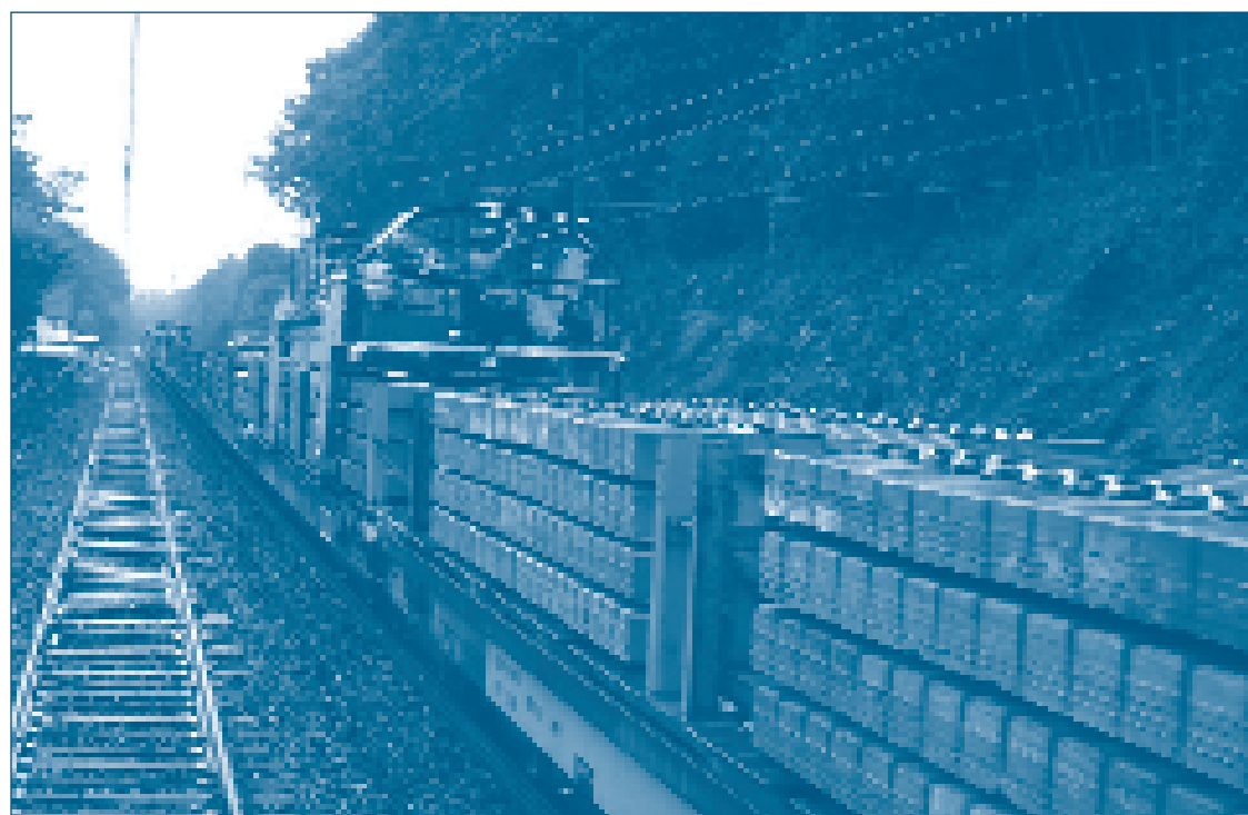
The concrete ties loaded on the distribution gantry of the Track Laying Machine make up some of the 128,000 ties laid on the Keystone Corridor over the course of 16 months.
