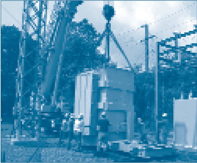
The Perryville substation crew moves a new transformer onto its base for permanent installation.
