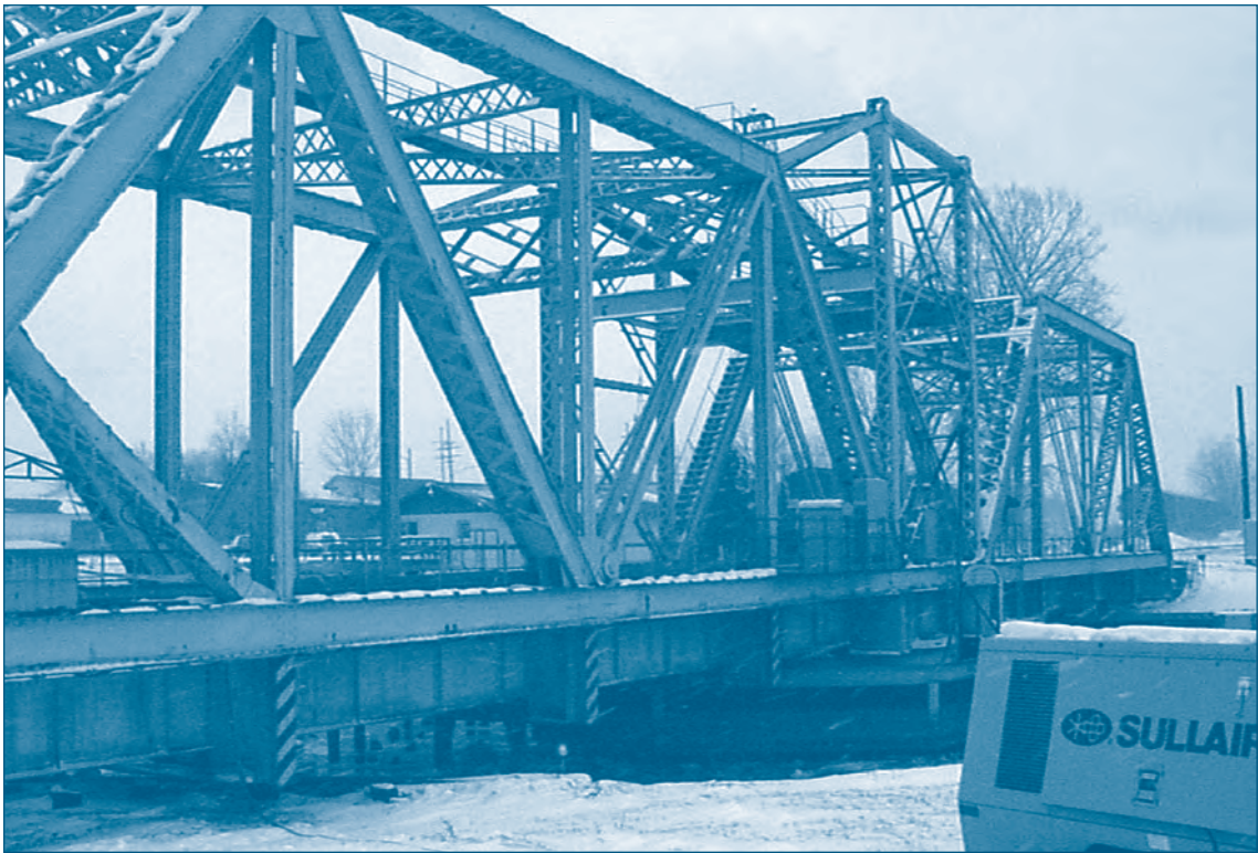
The Niantic River Bridge in East Lyme, CT, opens for marine vessel traffic. The bridge has been plagued by operating failures due to cracked steel girders and other structural problems.
