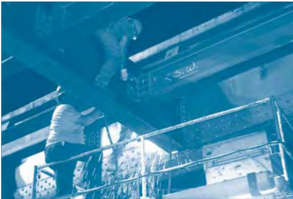
Jeff Thompson (L.) and Dave Settlemire install connection bolts at the stringer/floor beam connection.
