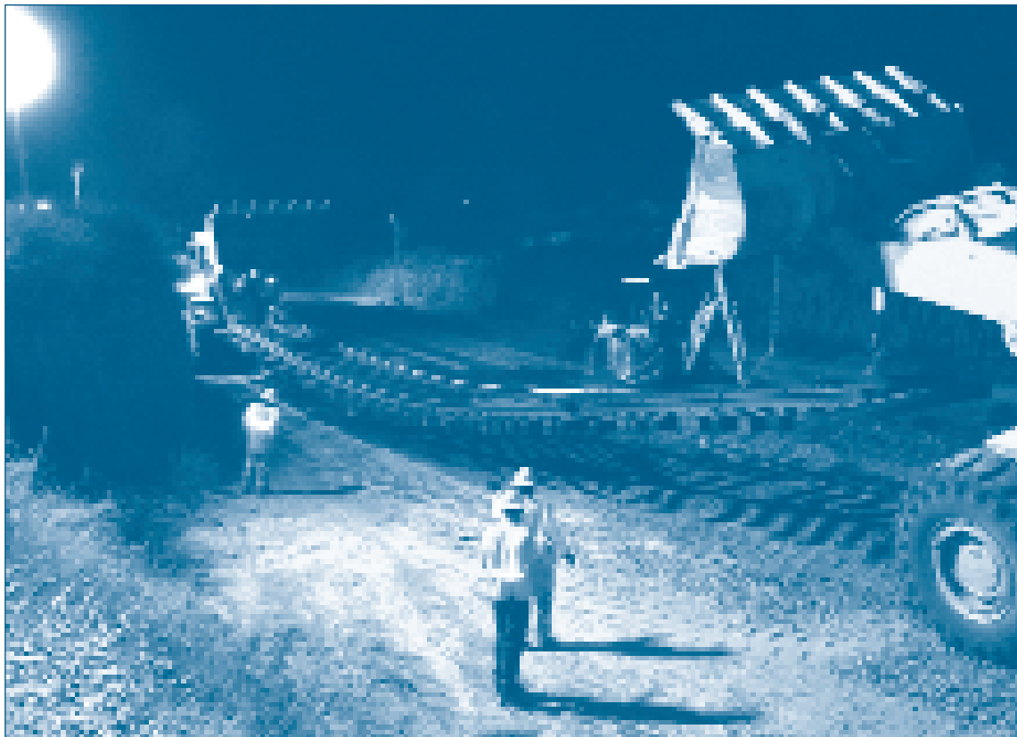
Track and Signal crews remove the old turnout at CP Ponto in Oceanside, Calif. Six endloaders and one excavator were used to remove and replace pre-built panels, and new signal cables were installed throughout the turnout. As a result of the replacement, trains can change tracks at 60 mph instead of 40 mph.
