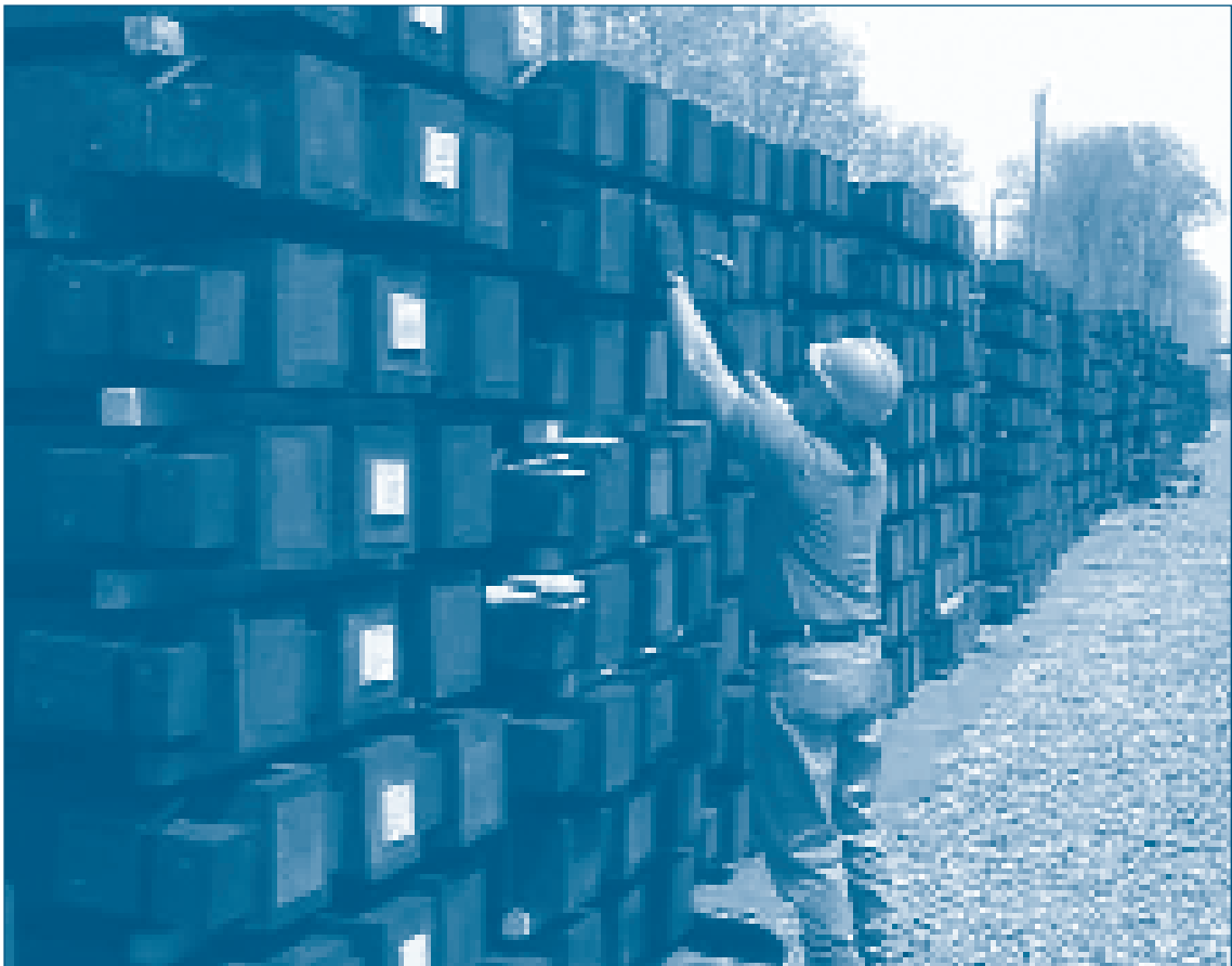
Bundles of more than 3,000 bridge ties that are slated for use in the Susquehanna River Bridge project are checked by Bridges and Buildings Mechanic Dave Settlemyre. The ties vary in size and are numbered according to their specific placement on the bridge.
