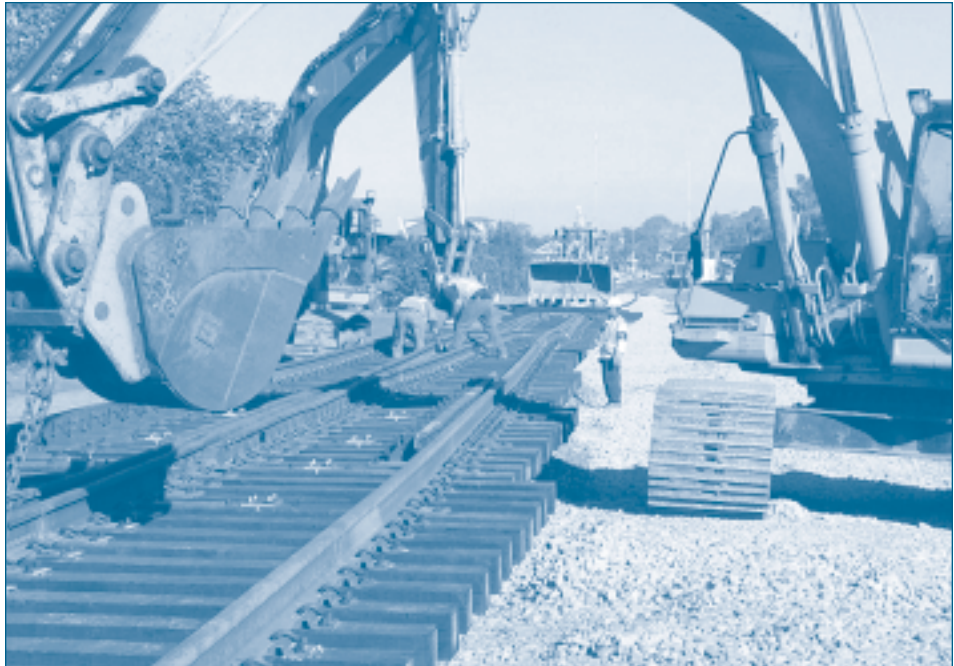
Crews install switch number 24 turn out on the SDNR in Encinitas, CA.
