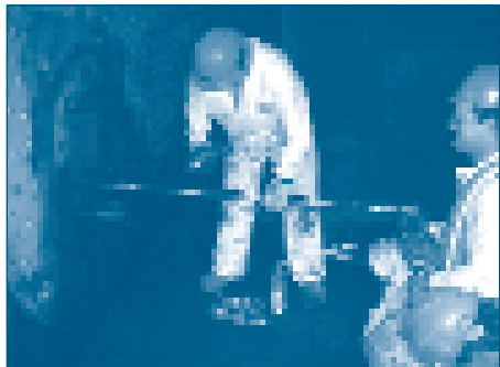
Engineering forces work around the clock to complete emergency repairs on the Thames River Bridge south counterweight trunnion. Broken bolts that were found during an inspection led to this weeklong effort.
