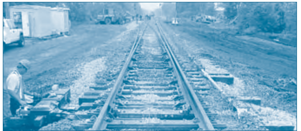
Signal Maintainer Jim Chaney completes the installation of a new switch while track employees distribute ballast and install new ties at Three Oaks.
