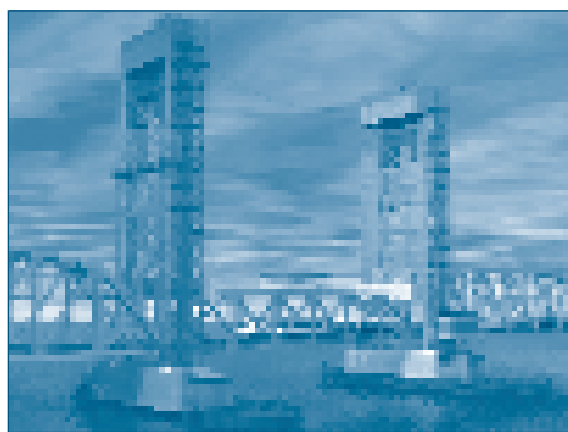
These graphic renderings of the new Thames River Bridge show the lift span lowered (left) for rail traffic and raised (right) to allow marine traffic to pass underneath. The work to replace the bascule span with the new lift span is expected to be complete the winter of 2007-2008.
