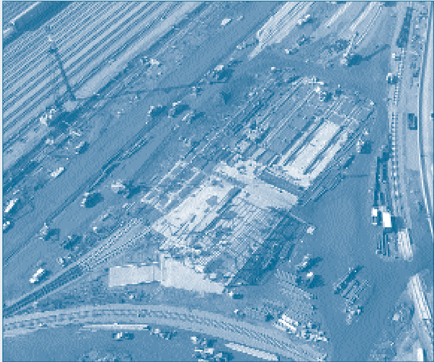
Construction on Amtrak's maintenance facility continues in Oakland, CA, with completion slated for the end of September 2004. The steel framing for the maintenance building is being installed, as well as construction of the service and inspection pit, and the wye East and wye West tracks. Currently, the $65-million facility is approximately 75 percent complete. Photo credit: William Hill
