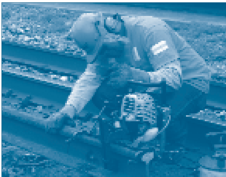
Machine Operator Freddie Butts, Jr. drills new bolt holes with a portable rail drill as part of the rail replacement program on the Harrisburg Line.
