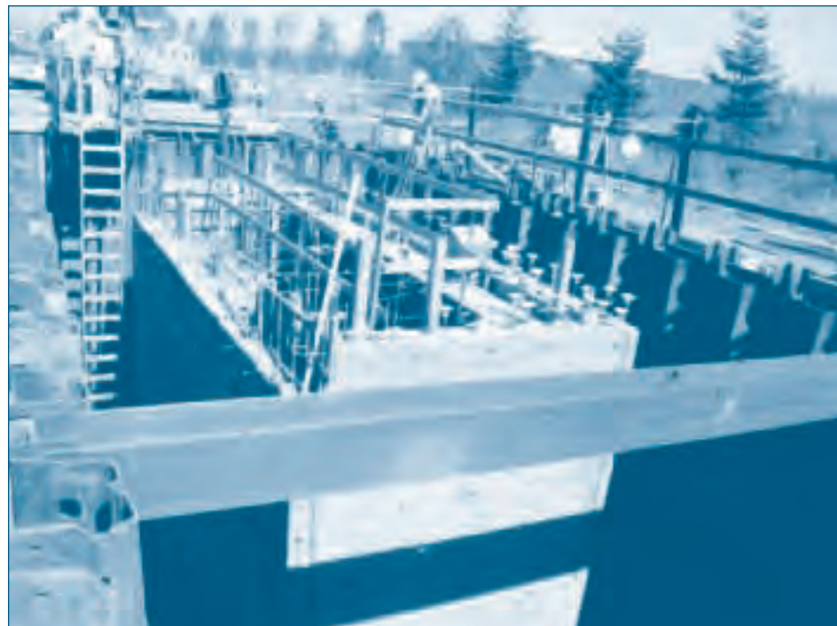
Workers pour concrete into the new trainwasher walls at the Oakland Maintenance Facility.
