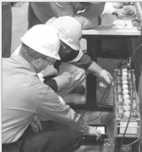
Communications and Signals Instructor Steve Bagosy shows Jason Foster the proper procedures for checking battery voltage.
