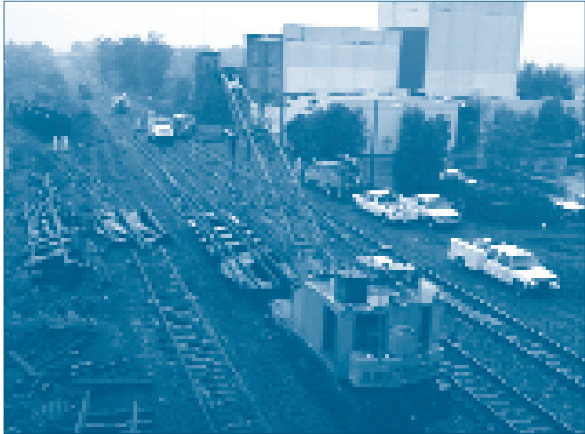
The Elm Interlocking in Greensboro was reconstructed to once again accommodate passenger trains at the historic Greensboro station. New crossovers were installed to enable trains to switch tracks at higher speeds.
