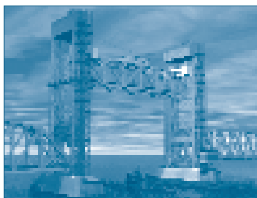
These graphic renderings of the new Thames River Bridge show the lift span lowered (left) for rail traffic and raised (right) to allow marine traffic to pass underneath. The work to replace the bascule span with the new lift span is expected to be complete the winter of 2007-2008.
