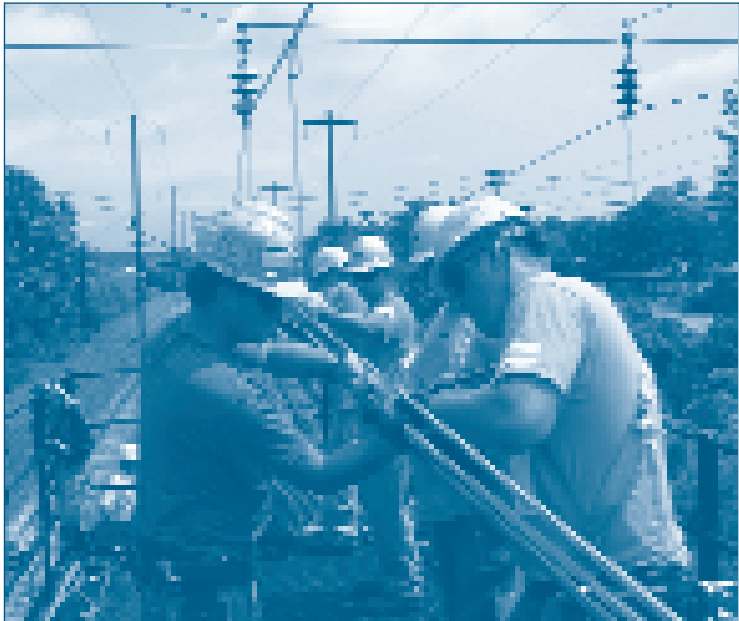
The Perryville electric traction crews pull the slack from the catenary trolley wire as they stand on the catenary maintenance vehicle hydraulic-lifted platform.
