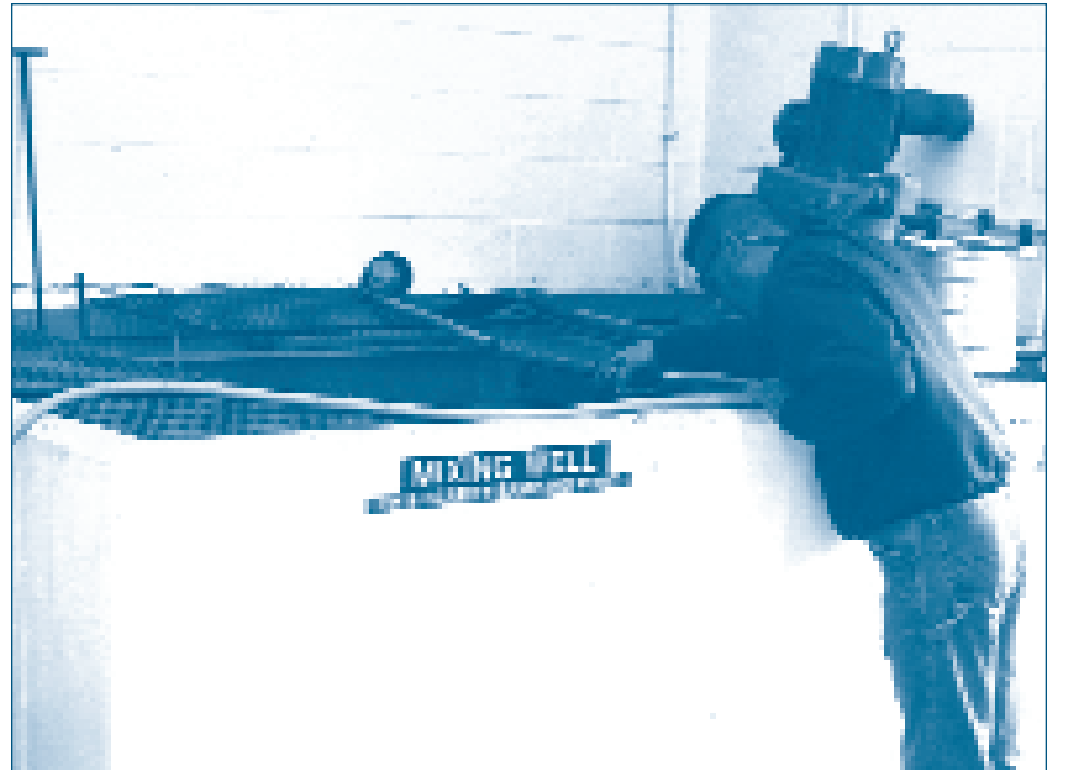
As a wastewater treatment operator, Christopher Lento (currently a Mechanical foreman III) monitors the mixing tank where chemical additions and pH adjustments are made to the wastewater prior to its transfer to the DAF system’s primary treatment tank.
