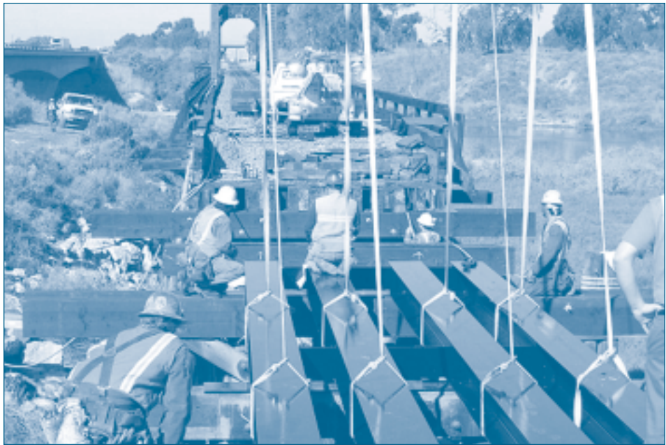
Crews replace four spans on SDNR bridge number 223 in Oceanside, CA.
