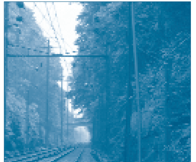
Overgrown trees and brush on the Harrisburg Line can cause power failures and service disruptions. The vegetation along the right of way in Conewago, PA, was one of the project's long-overdue targets.
