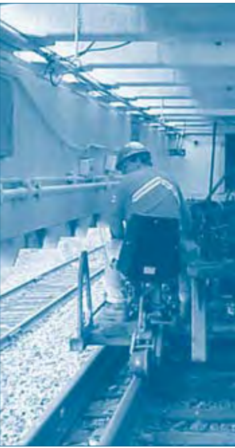
Counterclockwise from top left: Maintenance of Way employees, using the Burro crane, set up new rail in position for the TLM. TLS tie cars seen at a curve provide a partial perspective of the system consist length. From within the TLM, workers remove the spikes from the old wood ties.
