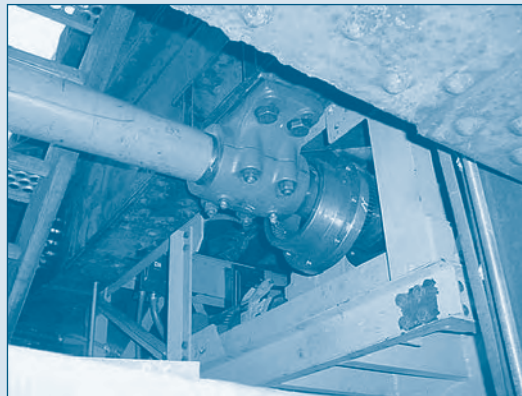
Updated machinery components, such as new bearing and shafts seen in this photograph, provide a temporary solution to the Niantic River Bridge's malfunctions.
