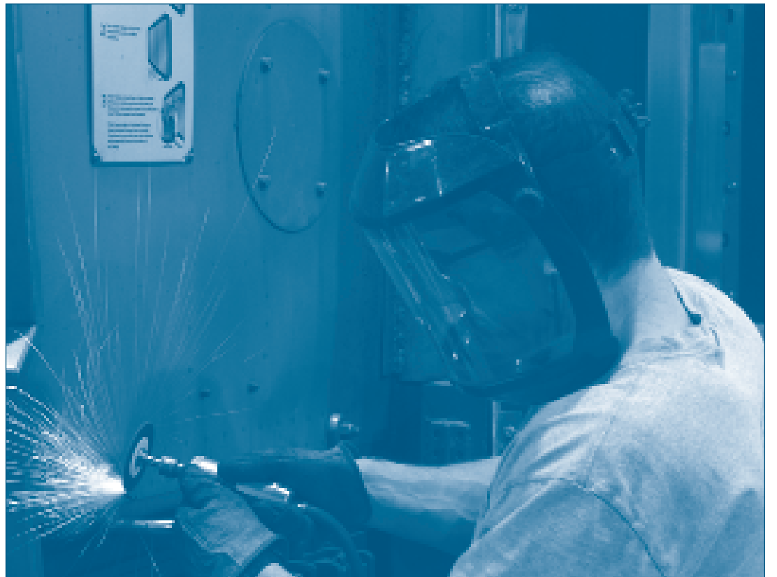
Car Repairman/Welder J. Bruce Carlton installs a grab iron on cab car 9646 at Bear Car Shop. The grab iron is a safety feature used by the crews to hold on to when pulling cables or coupling the train.
