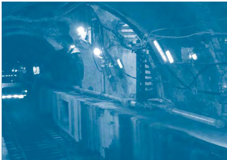
The fire standpipe work in progress in the East River Tunnel contributes to the goal of installing a total of 16 miles of standpipe in all six Amtrak tunnels.
