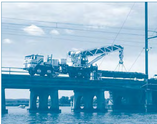
The Gunpowder River Bridge is a critical link between Wilmington and Baltimore on the Northeast Corridor. Decayed wood timbers and deteriorated steel beams were replaced with concrete.
