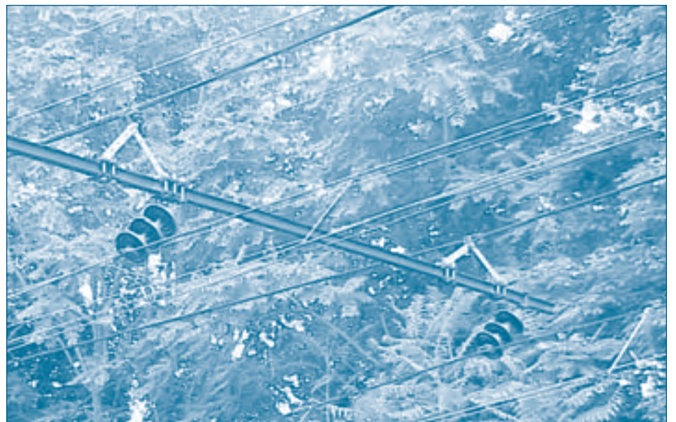
This suspended (floating) catenary on the Hell Gate Line has been in service since the early 1930s.
