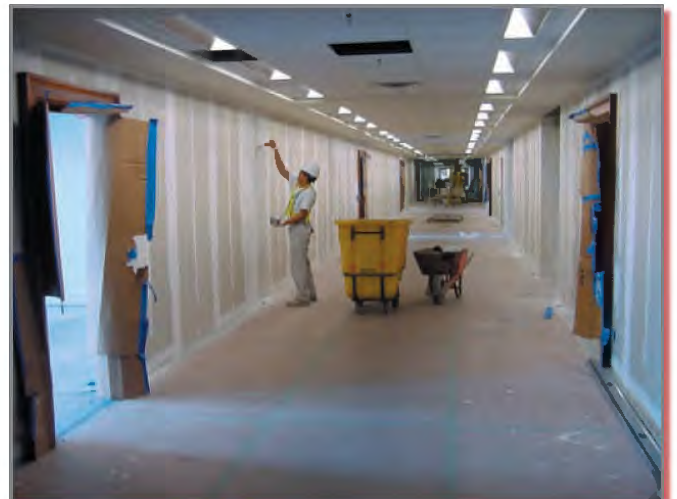
A construction worker finishes an E ring wall.
